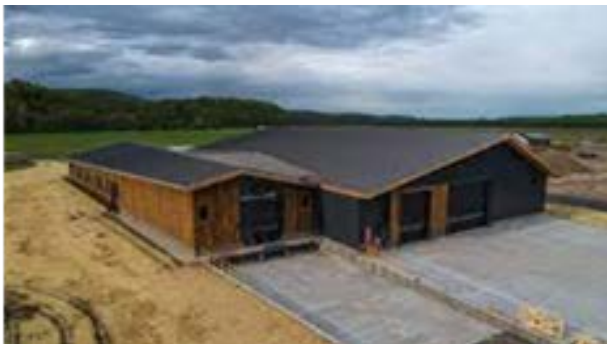
Examples of desirable building types for light industrial uses
