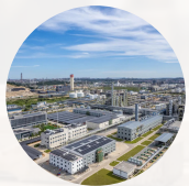
Factory Setup & Infrastructure Development
