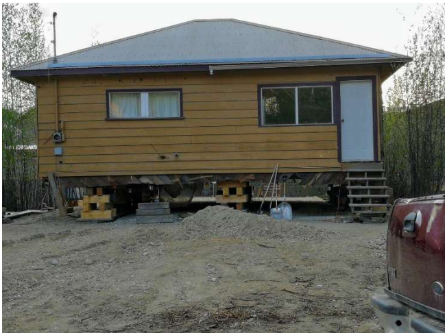
Figure 6. An image of a house in Dawson City, Yukon. Buildings are constructed on raised supports to minimize heat transfer from the home to the ground and slow permafrost thaw. Deep foundations help to keep the home stable and prevent it from sinking into the ground as global temperatures rise and permafrost thaw worsens.
