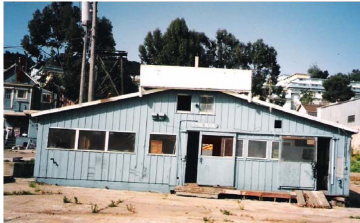
Figure 4. Anderson & Cristofani Boat Yard Compressor House & Paint Shop
