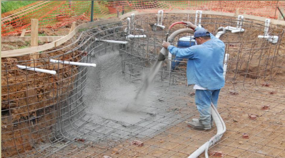
Paddock was the first company to use gunite, a term used to describe pneumatically applied concrete. Before gunite, pool builders would use traditional poured in concrete,
