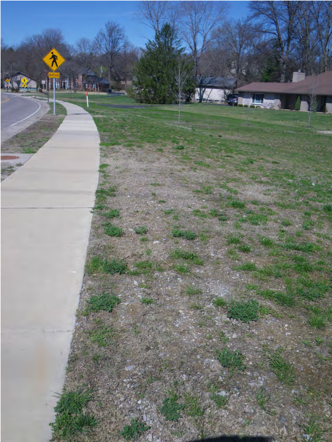
Village of Green Trails Entrance: Rock left from intersection construction prevents grass from growing.
