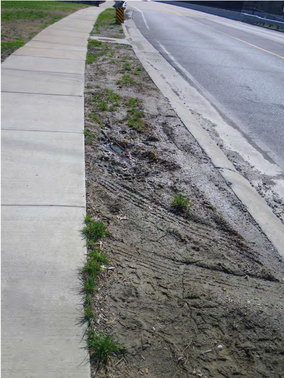
Ruts are caused by trucks driving over the N entrance grounds to access VGT grounds S of Ladue Rd.
