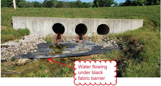
2. Due to major storms, the downstream channel's rock revetment (similar to the rock on the banks) has been washed away with portions of the black fabric barrier. The earth is exposed and susceptible to erosion, deep cutting, and meandering of the channel.
