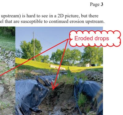
3. The next two pictures below (looking upstream) is hard to see in a 2D picture, but there are two significant drops in the channel that are susceptible to continued erosion upstream.
