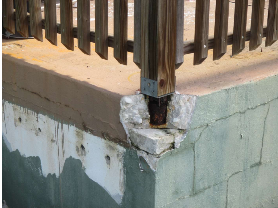
Photograph 17 South Façade Entry Handrail - Base Deterioration
