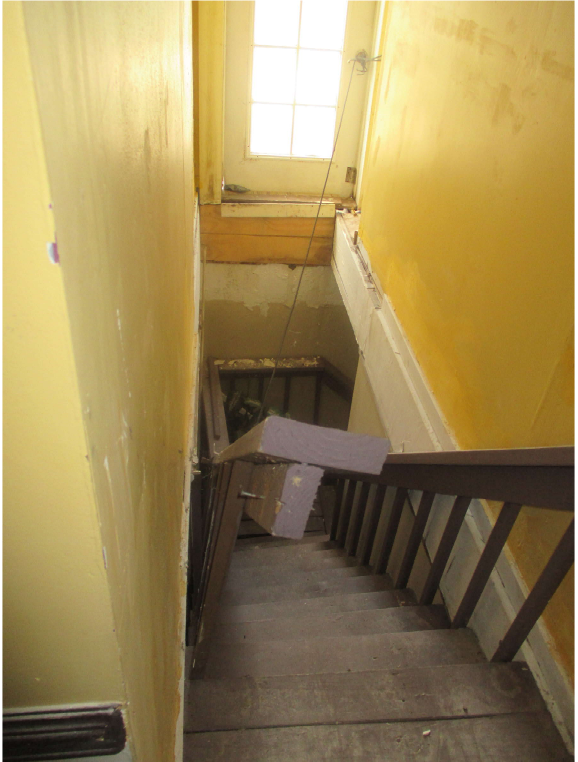
Photograph 11 Failed Stairs and Handrail at Northeast Corner
