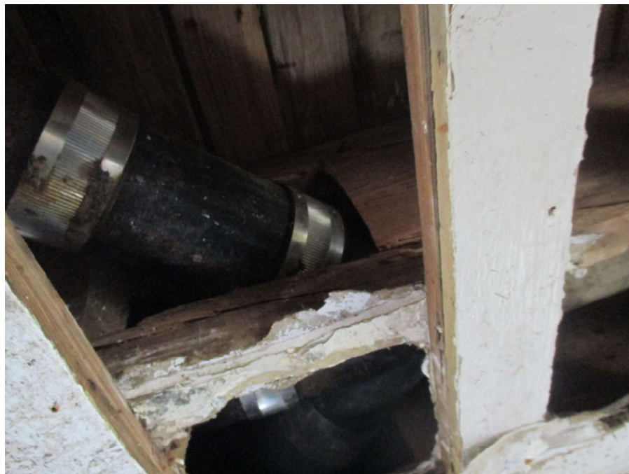
Photograph 10 Compromised Joist Due to Coping and Leaking Drainpipe
