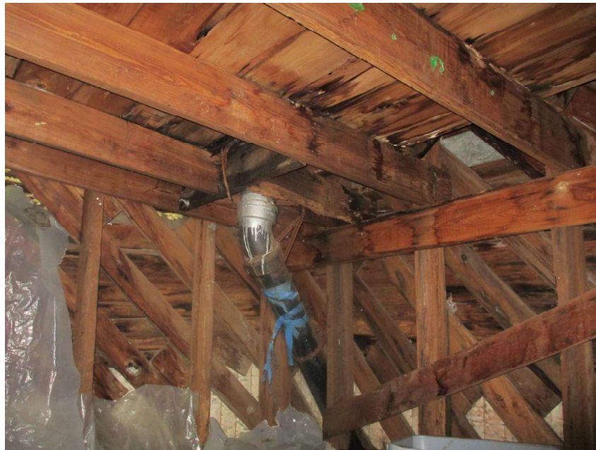
Photograph 4 Deteriorated Roof Framing at Drain
