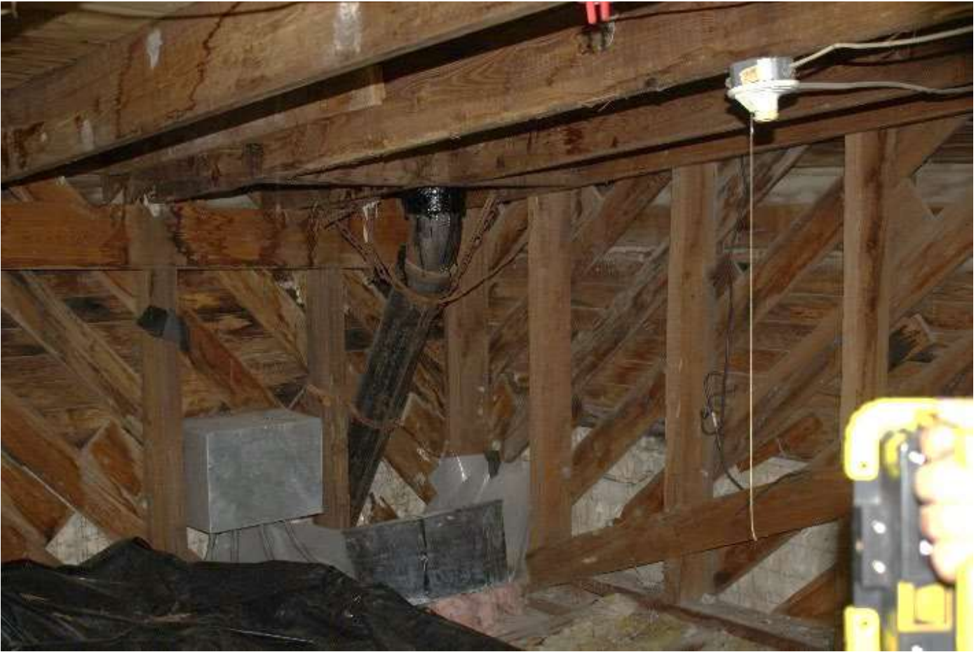
Attic area showing roof drain and plastic
