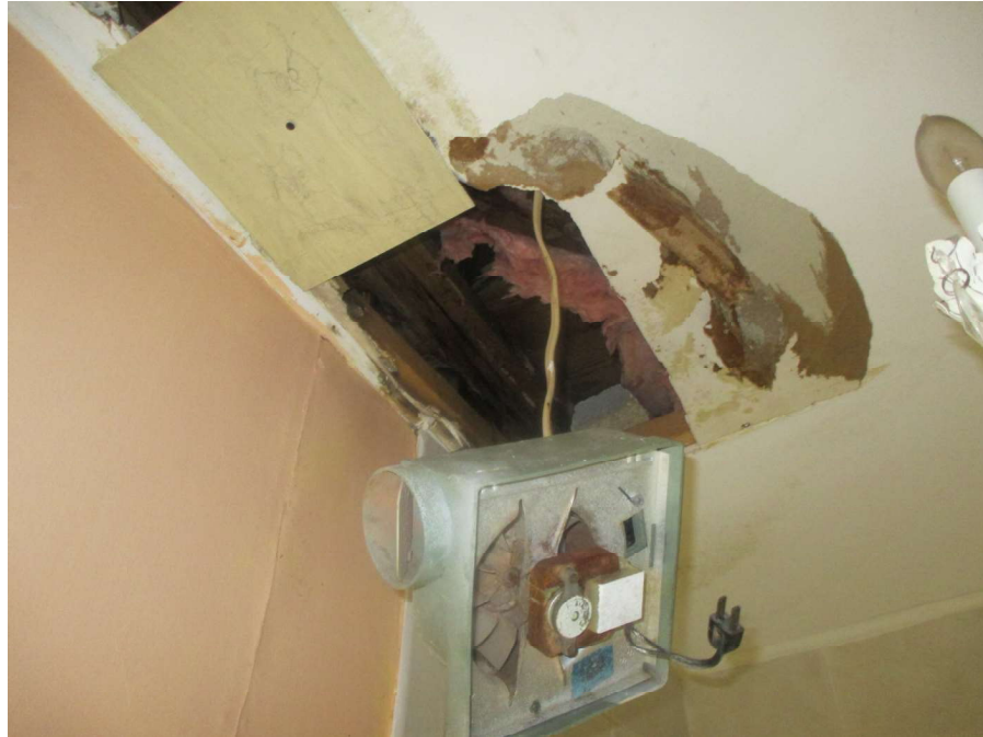
Photograph 9 Water Damaged Framing at Exhaust Fan
