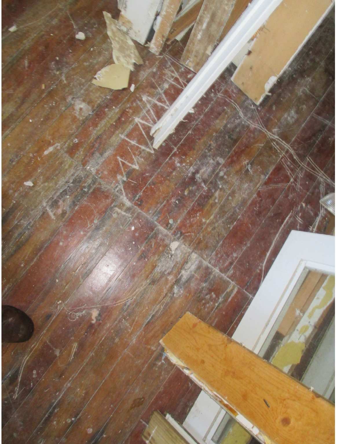
Photograph 12 Deteriorated First-Floor Decking
