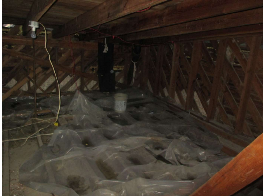
Photograph 5 Plastic Membrane in Attic Over Ceiling
