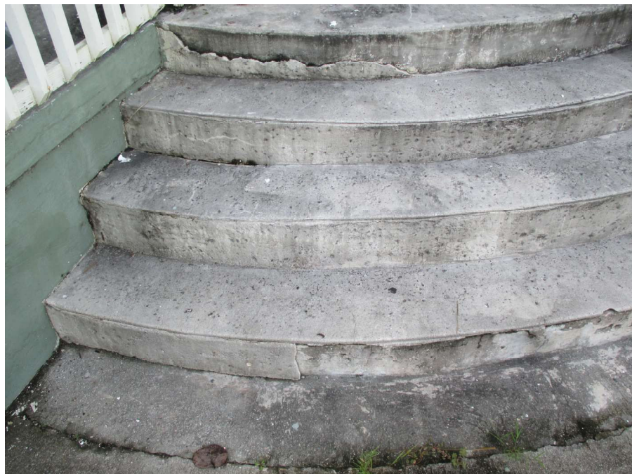
Photograph 16 West Façade Entry Steps - Topping Deterioration
