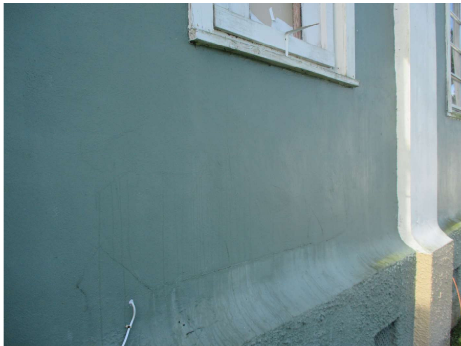
Photograph 20 Cladding Crack at First Floor Joint
