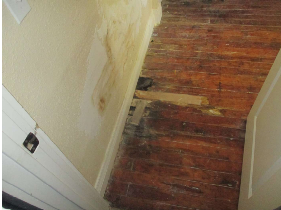
Photograph 7 Water Damage Due to Plumbing Leak
