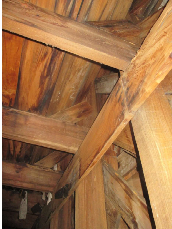
Photograph 3 Parapet Knee Brace
