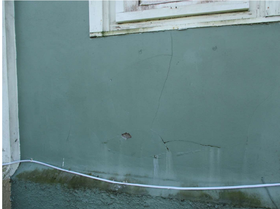
Photograph 19 Northwest Corner Cladding Spall
