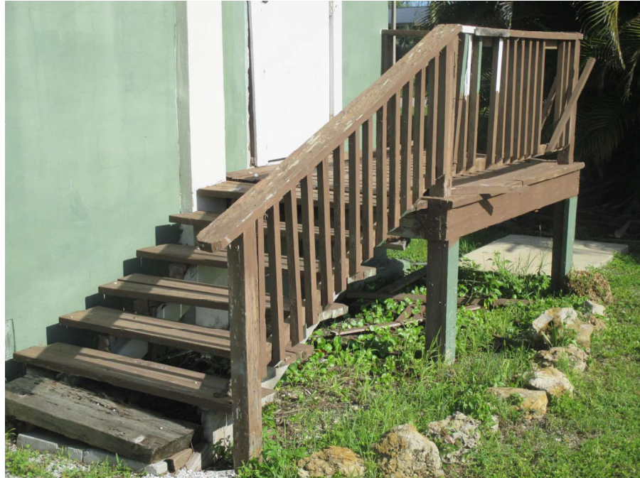
Photograph 15 Failed Handrail and Bearing On Grade
