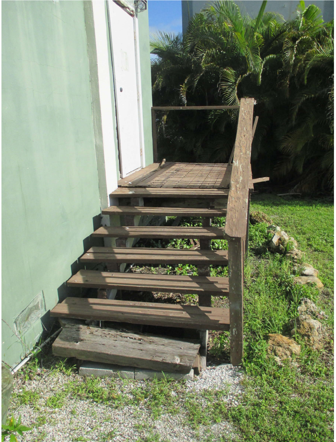
Photograph 14 East Facade Deteriorated Wood Stair Requiring Replacement on New Footings
