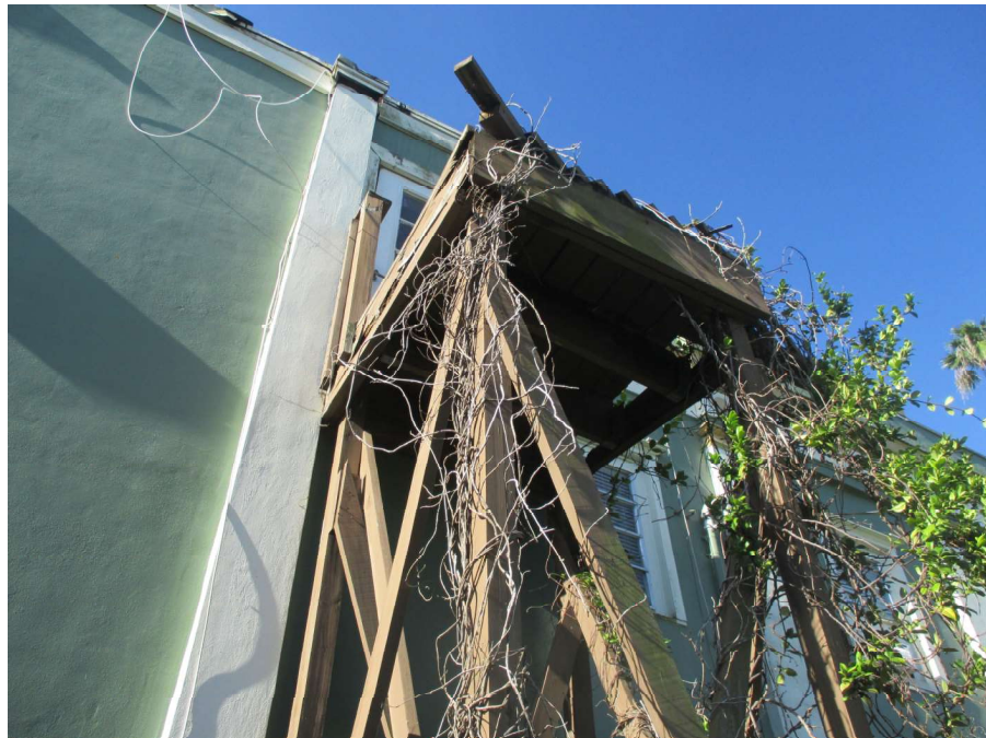
Photograph 18 North Façade Entry Deterioration
