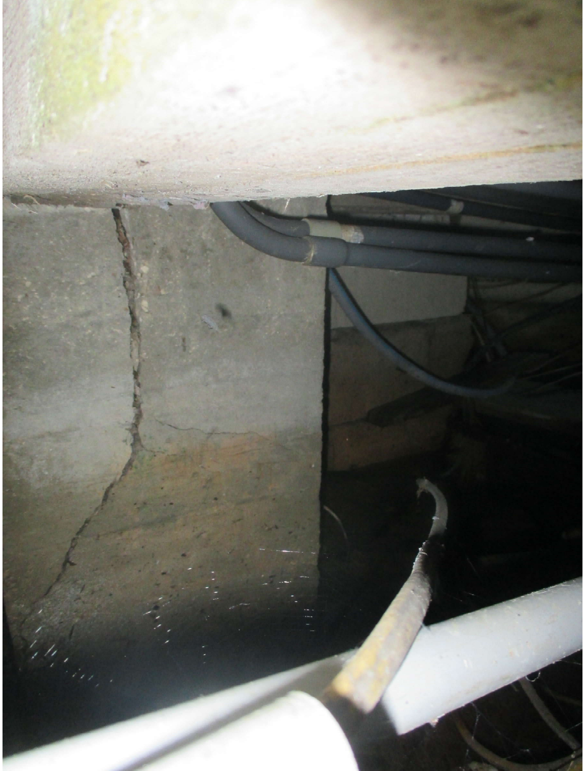
Photograph 13 Northeast Foundation Pier Cracked
