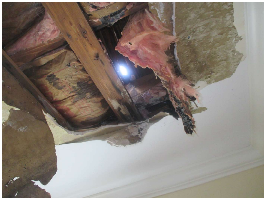
Photograph 6 Rear Addition Low Roof Opening
