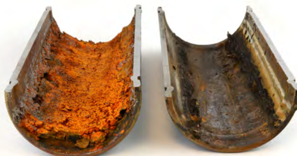
20 Month Pipe Test with Air
