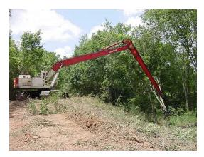
c). The COE requires that all stumps be left in the banks to prevent erosion. The grapple saw cuts the trees and leaves the stumps at about 6 in tall.
