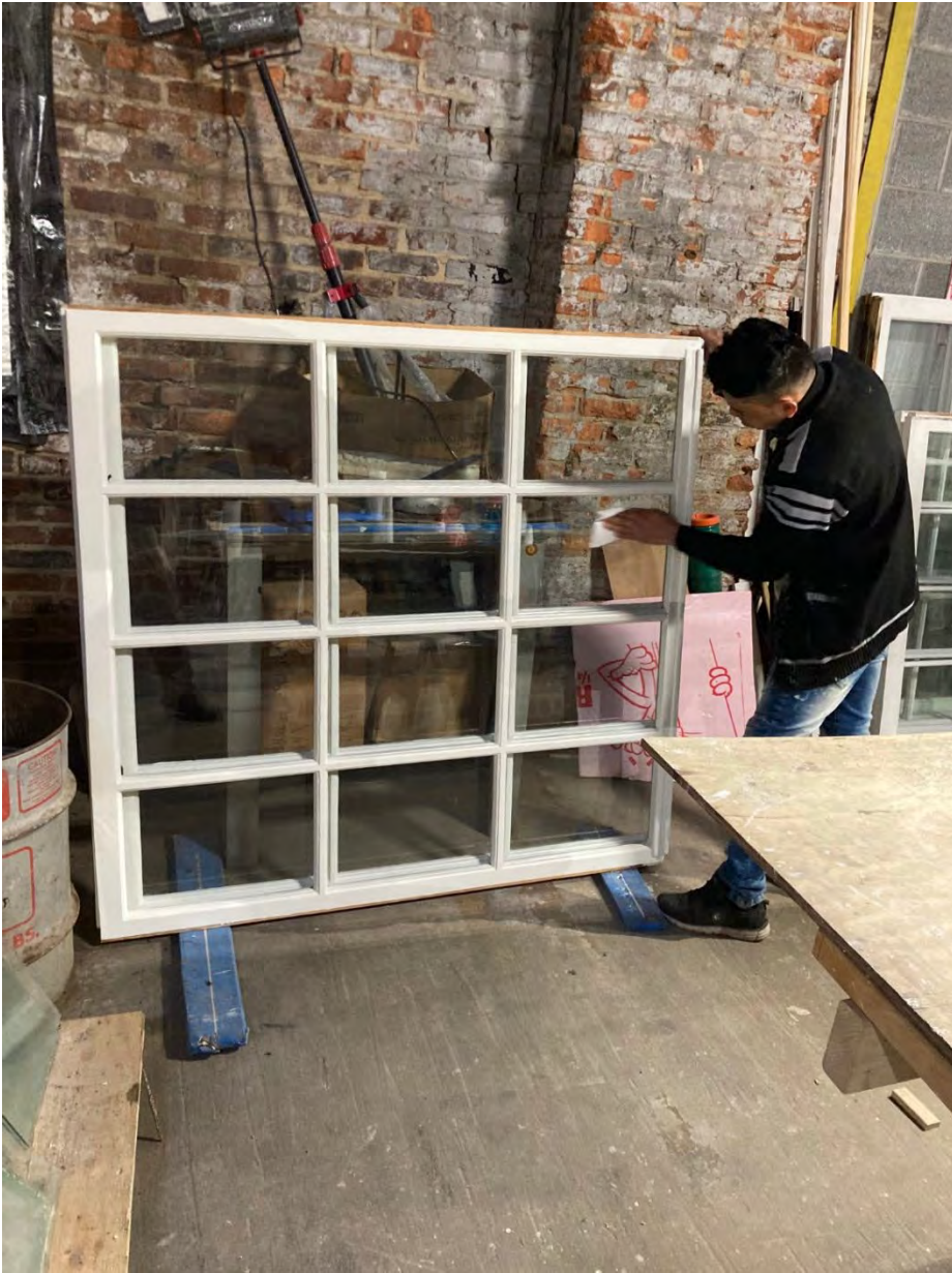
Restoration of windows from Hopkins Latrobe Hall. Each sash is five feet tall and four feet wide with 12 lites.
