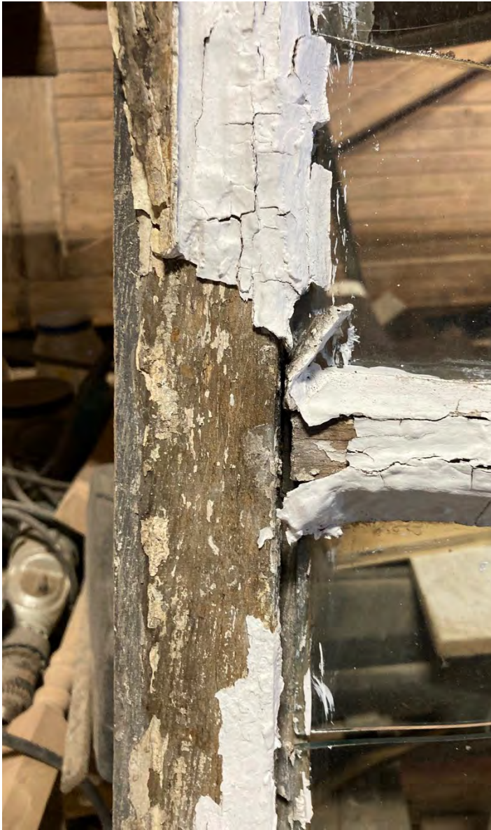
In-process restoration of windows from Hopkins Latrobe Hall. Each sash is five feet tall and four feet wide with 12 lites.
