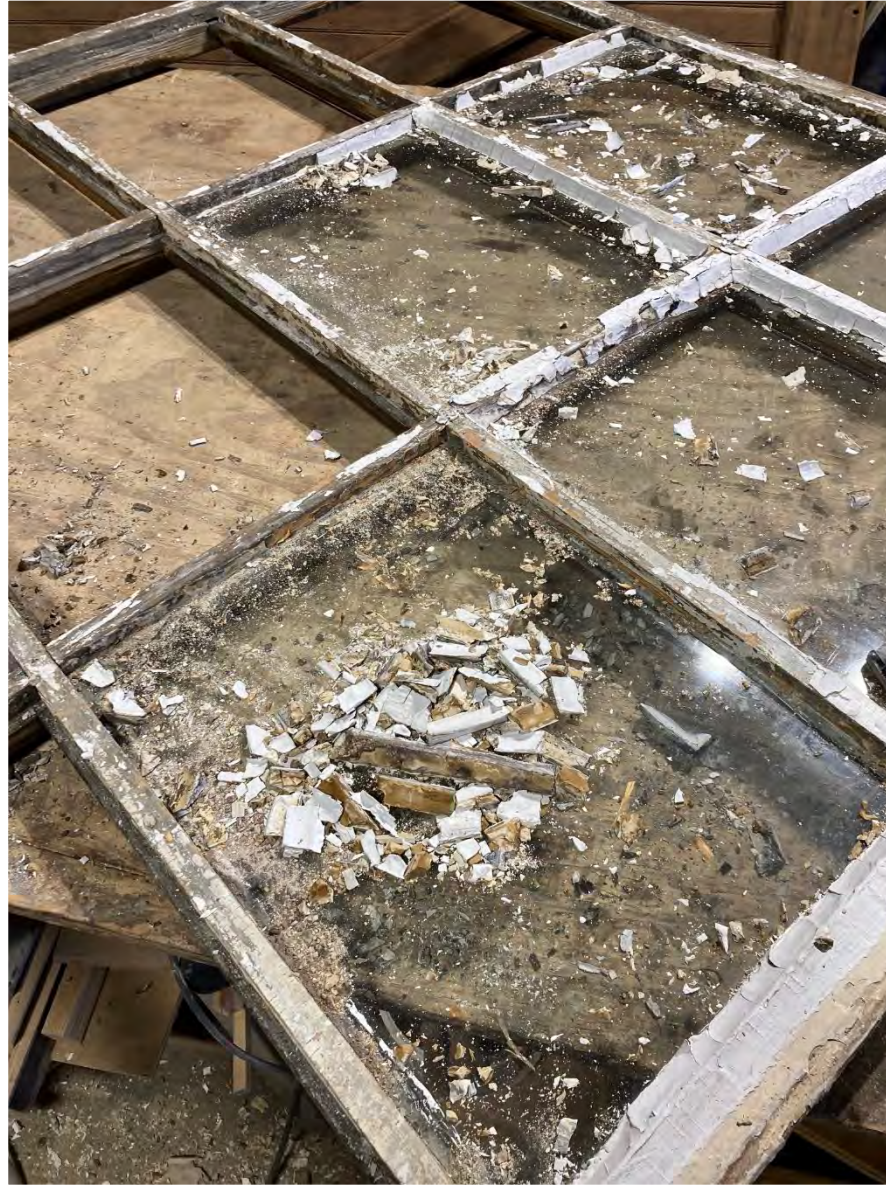
In-process restoration of windows from Hopkins Latrobe Hall. Each sash is five feet tall and four feet wide with 12 lites.
