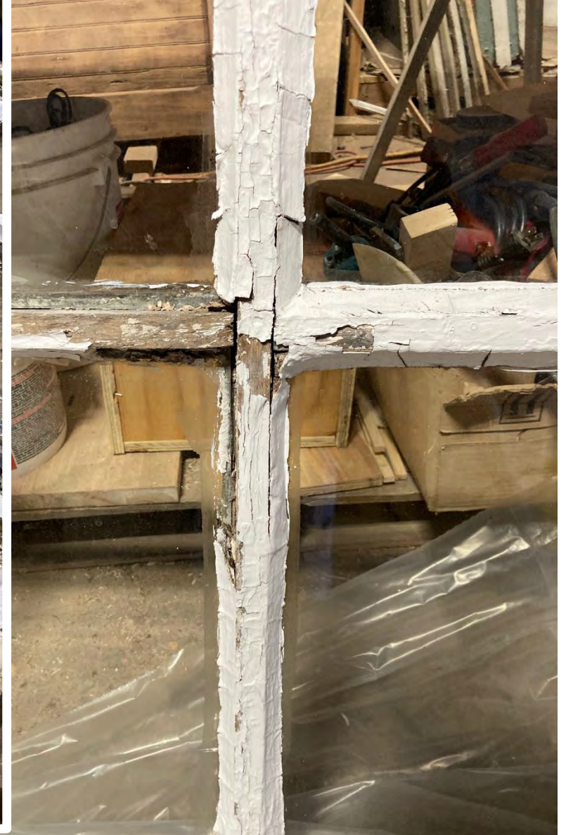
In-process restoration of windows from Hopkins Latrobe Hall. Each sash is five feet tall and four feet wide with 12 lites.
