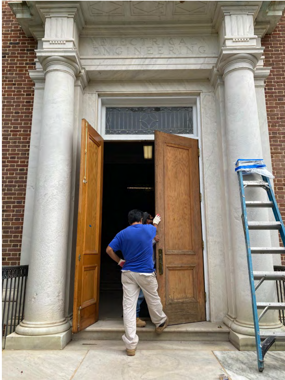
In-process and after (on right) photos of restored water damaged mahogany doors at Hopkins Homewood Campus Maryland Hall.
