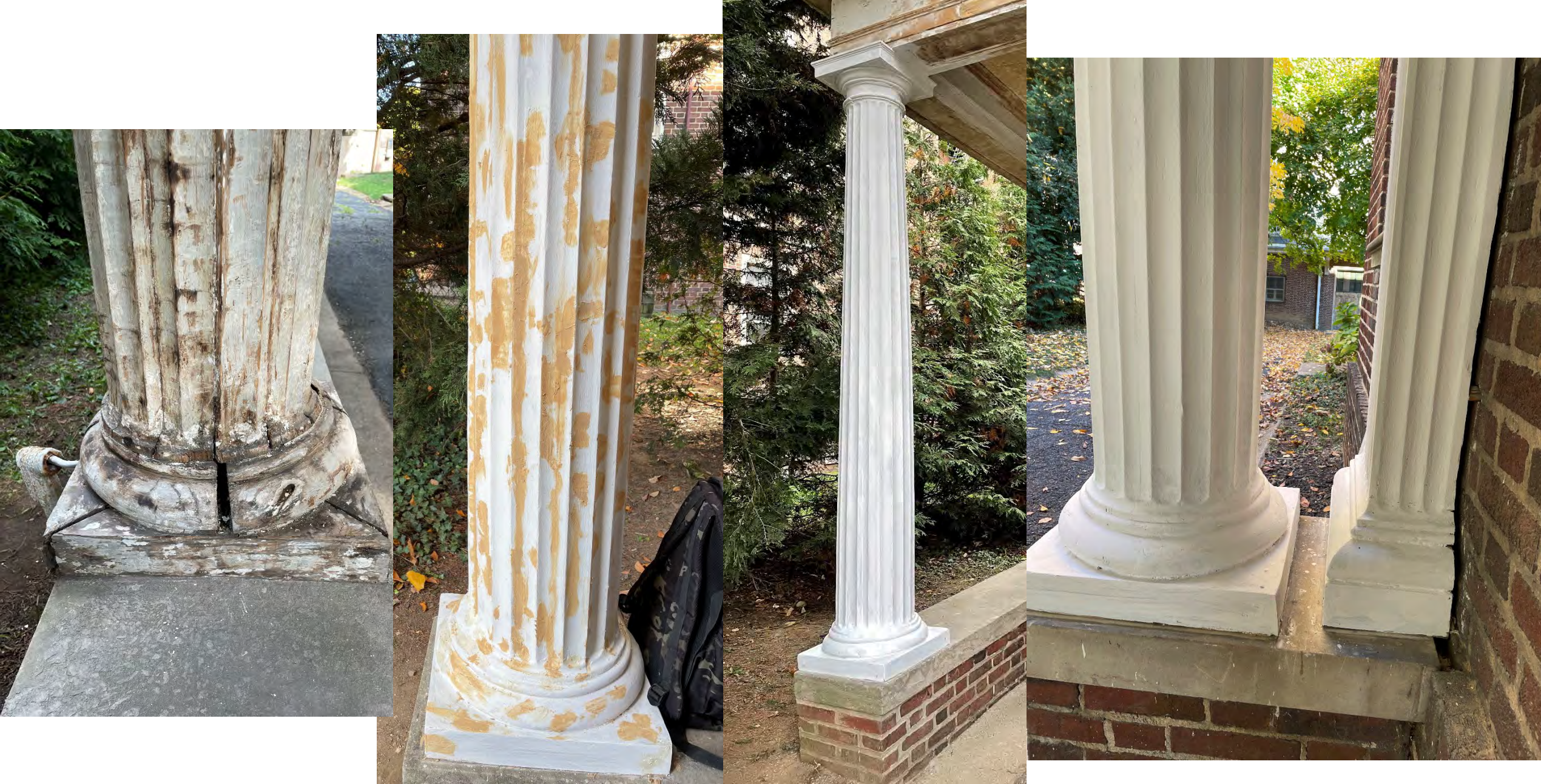
Before and after photos at 3505 N. Charles Street showing repaired and restored portico columns.
