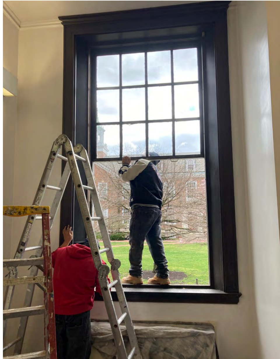
Restoration of windows from Hopkins Latrobe Hall. Each sash is five feet tall and four feet wide with 12 lites.
