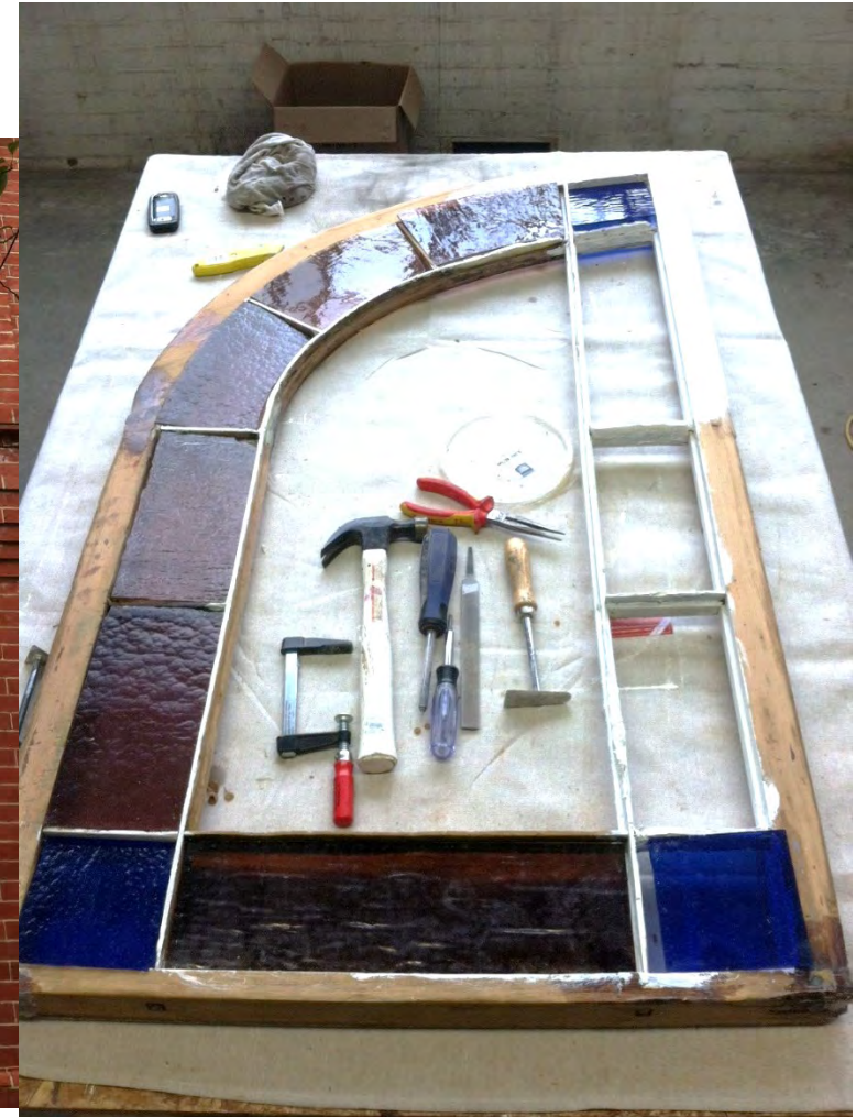
Wood window restoration of 12 foot high original wood windows with stained glass repairs, 1809 St Paul Street, Baltimore, MD. Building built circa 1880.
