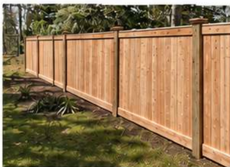
Finished Cedar Trim
