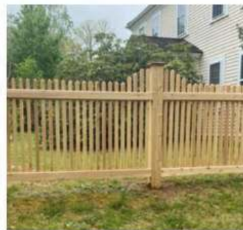
Clean Fascia Finish
