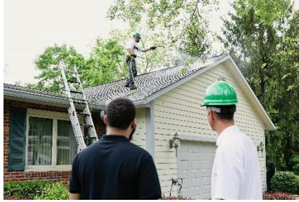
Property owners have an eco-friendly and much less expensive alternative to roof replacement. In a nutshell, it is a shingle rejuvenator in the form of a sustainable plant-based spray that when applied to existing shingles that can extend the life of asphalt roofs by five years per treatment. By repeating the process every five years, a property owner can extend a roof's life by as much as 15 years for around 15% to 25% the cost of replacement.
