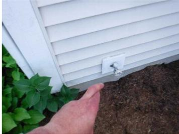
Maintenance/Improvements: Vents: Dryer vent extends out excessively. Recommend repair.
