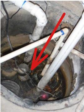
10. Main Basement Radon Unit: The radon unit was not functional at the time of inspection. The radon discharge was too low and should discharge 8 feet above ground level. Recommend repair by a qualified contractor.
