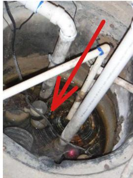
Maintenance/Improvements: Radon Unit: The radon unit was not functional at the time of inspection. The radon discharge was too low and should discharge 8 feet above ground level. Recommend repair by a qualified contractor.
