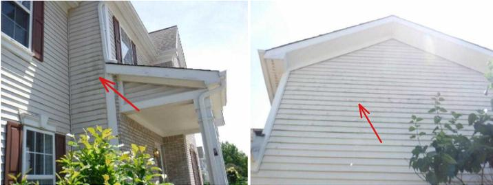
4. Vents: Dryer vent extends out excessively. Recommend repair.
