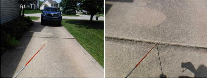
2. Steps/Stoops: Non conforming step risers. Trip hazard. Recommend repair/replace by a qualified contractor.
