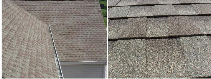
Maintenance/Improvements: **Flashing:** No flashing (edge/snow guard) installed from roof to gutters, prone to possible leaks and fascia damage due to ice damming. Recommend install flashing. (see graphics for example of proper flashing.)
