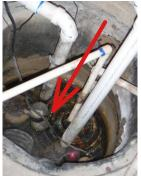
Maintenance/Improvements: Radon Unit: The radon unit was not functional at the time of inspection. The radon discharge was too low and should discharge 8 feet above ground level. Recommend repair by a qualified contractor.
