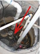
10. Main Basement Radon Unit: The radon unit was not functional at the time of inspection. The radon discharge was too low and should discharge 8 feet above ground level. Recommend repair by a qualified contractor.
