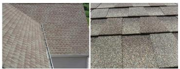
Maintenance/Improvements: Flashing: No flashing (edge/snow guard) installed from roof to gutters, prone to possible leaks and fascia damage due to ice damming. Recommend install flashing. (see graphics for example of proper flashing.)
