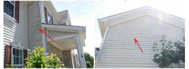
4. Vents: Dryer vent extends out excesively. Recommend repair.
