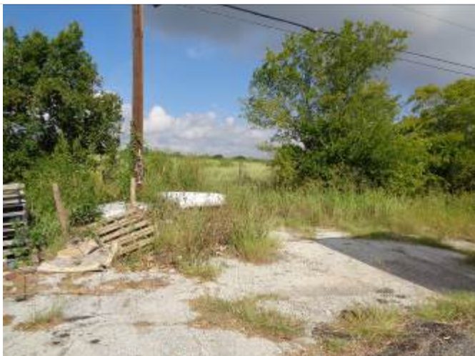
14. Terminus of Profit Centre Drive on the southeastern corner.
