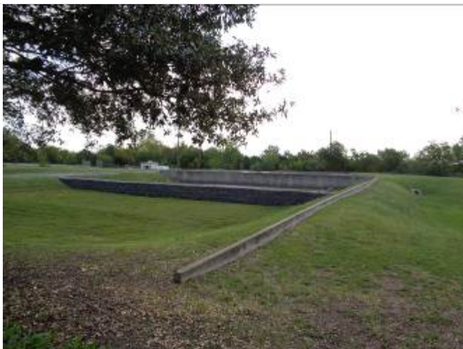
24. Another stormwater quality pond on properties to the west.
