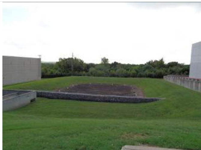
23. Stormwater quality ponds on adjoining properties to the west.
