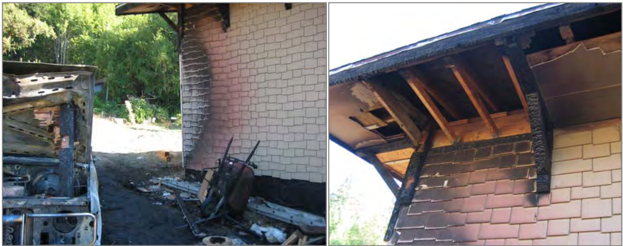
Photo 4-1: The photos above show damage that took place to a rural West County home when the vehicle on the far left ignited (cause undetermined). Highly aware of the wildfire risk in their area, the homeowners had recently replaced wooden siding with fiber-cement shingles, and enclosed the soffit with fiber cement sheathing. They also have well-maintained defensible space. The fire burned for at least one-half hour before firefighters were notified and arrived on the scene. Due to intense heat from the vehicle, there was some fire intrusion into the attic space which had to be repaired. However, if the residents had not taken action to replace flammable siding, it is likely that the home would have been a total loss. Likewise, their good defensible space kept the fire from spreading into the surrounding wildland.
