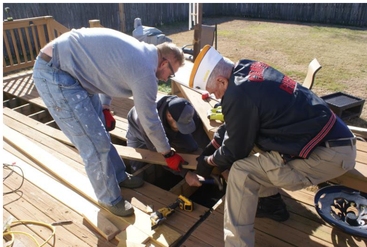
Volunteers work together to repair deck boards on the Bullard residence.
