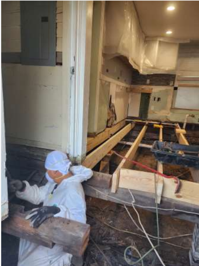
Volunteers work on the foundation to Ms. Caldwell's home.
