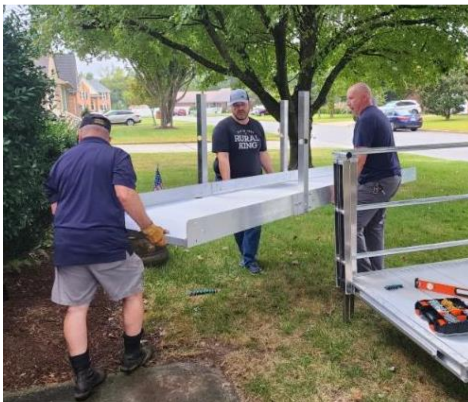
Volunteers from VFW Posts 2582 and 2894 place aluminum ramp sections during the construction of a wheelchair ramp for a Vietnam veteran and his wife in Suffolk, Virginia.
