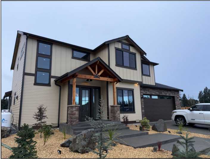
Missing address numbers on the home which is required for final county inspection. (Fire Safety Concern)
