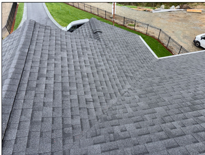
Roof – No Major Concerns
