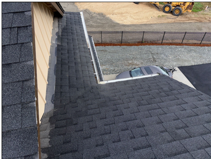
Roof – No Major Concerns
