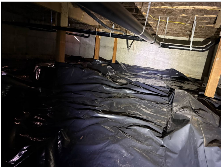
Vapor barrier present and appears to be properly installed.
