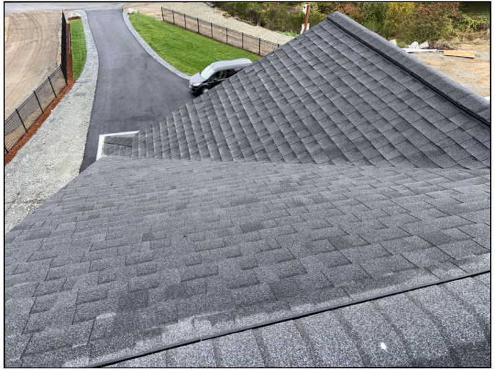
Roof – No Major Concerns
