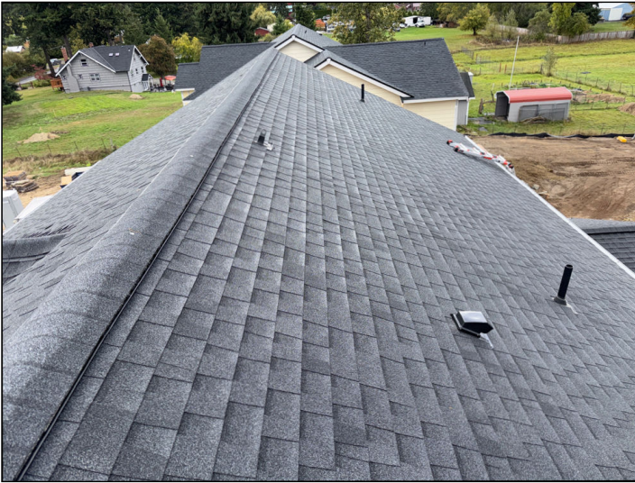
Roof – No Major Concerns
