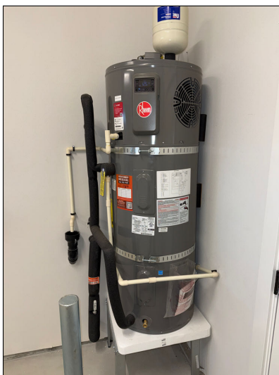
Seismic strapping present.
