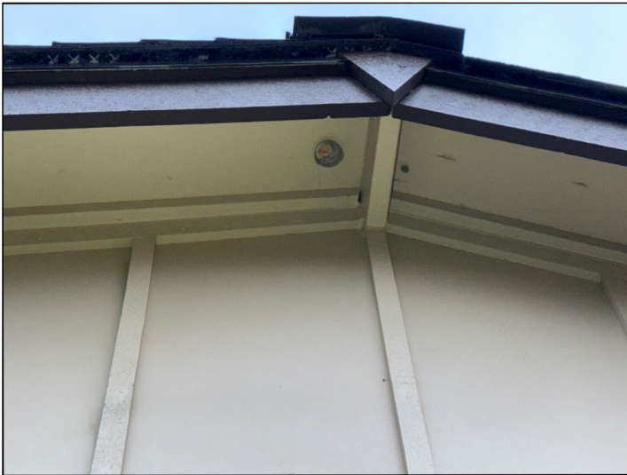
Paint touch up at the back patio gable / eave where a bees nest block full coverage and exposed plywood is present.
