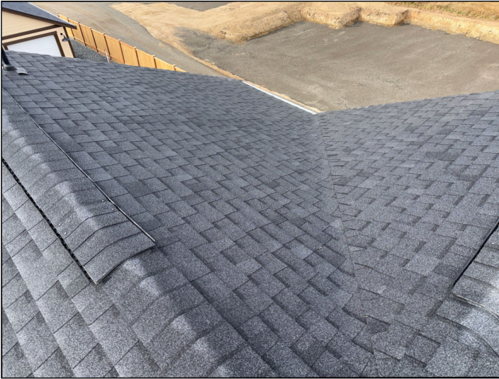
Roof – No Major Concerns
