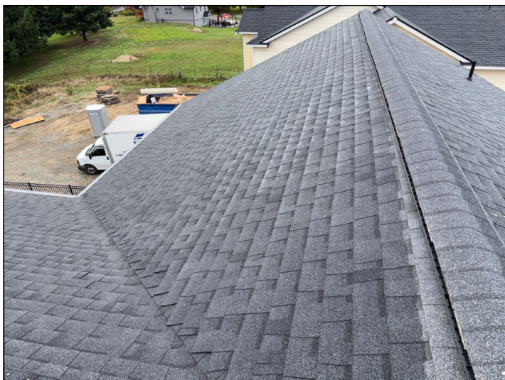
Roof – No Major Concerns
