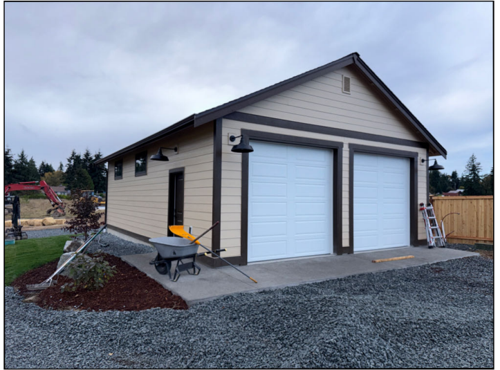
Appeared satisfactory, at time of inspection.
