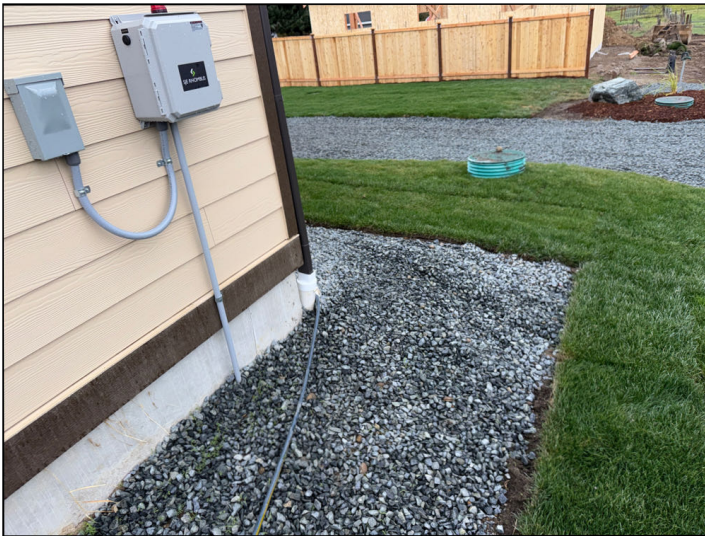
Septic clean out and tanks were noted on the South exterior side of the detached garage.
