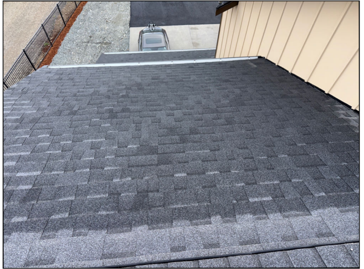
Roof – No Major Concerns
