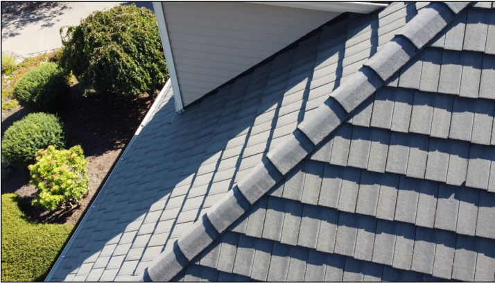
Roof – No Major Concerns
