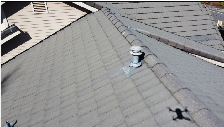
Roof – No Major Concerns
