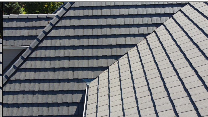
Roof – No Major Concerns
