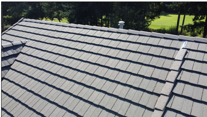
Roof – No Major Concerns
