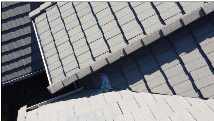
Roof – No Major Concerns
