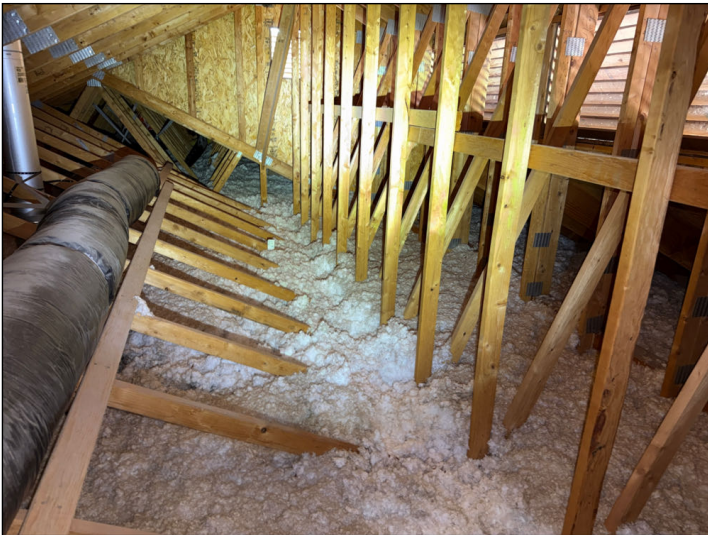
Insulation appears adequate and in good condition.
