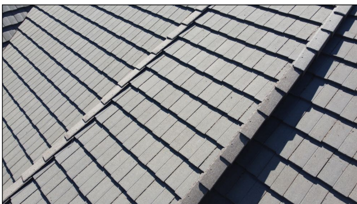
Roof – No Major Concerns
