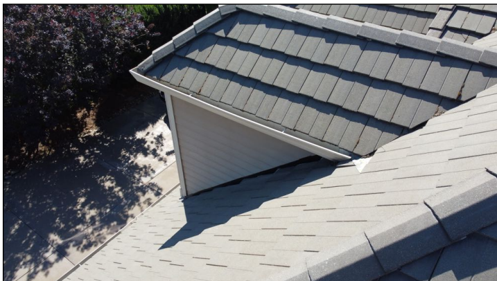
Roof – No Major Concerns
