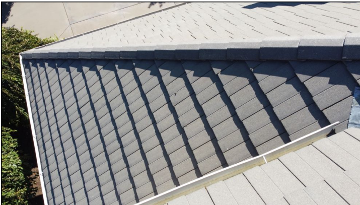
Roof – No Major Concerns
