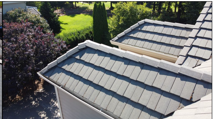
Roof – No Major Concerns
