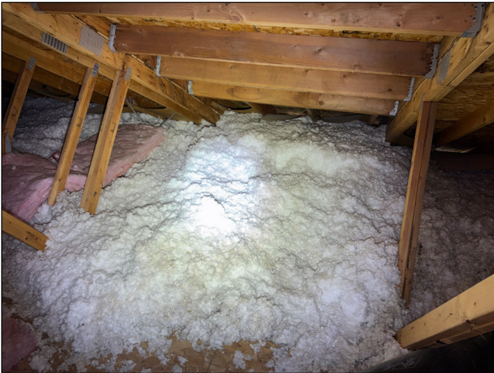
Insulation appears adequate and in good condition.
