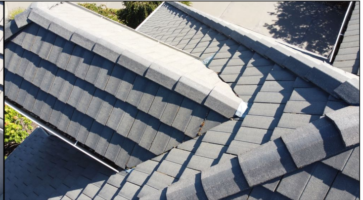
Roof – No Major Concerns
