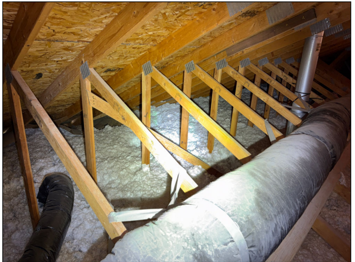
Insulation appears adequate and in good condition.
