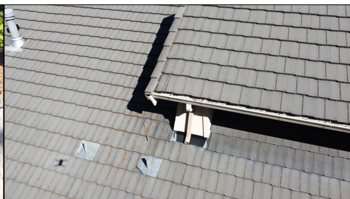
Roof – No Major Concerns
