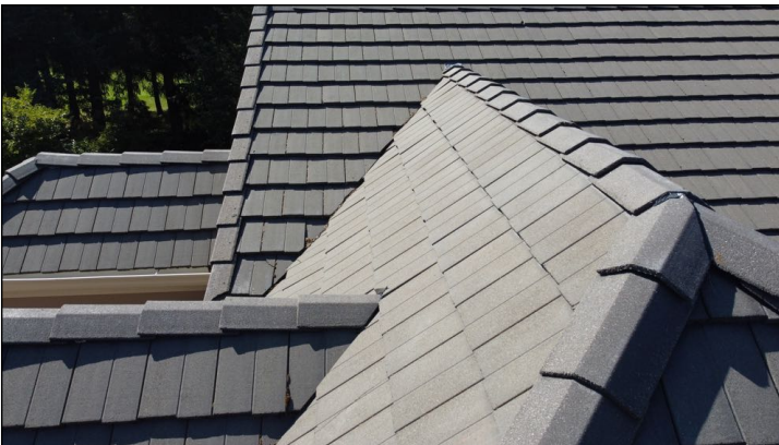
Roof – No Major Concerns
