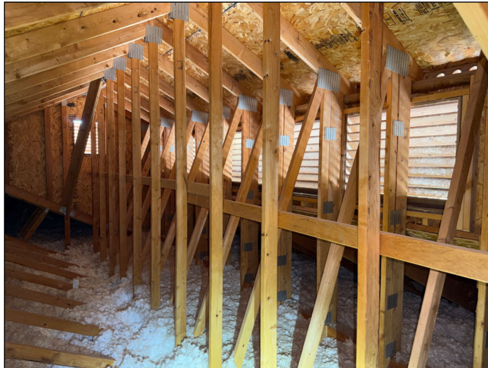
Gable louver vents noted.
