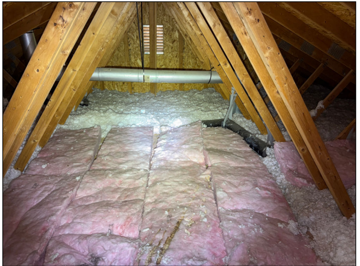
Insulation appears adequate and in good condition.
