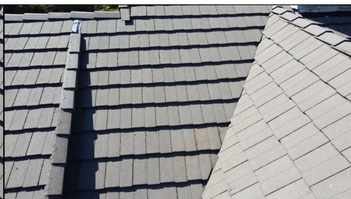
Roof – No Major Concerns
