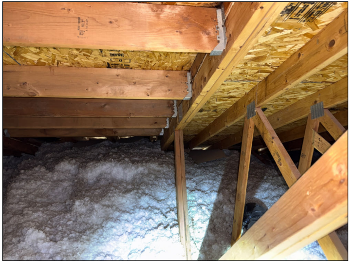
Under eave soffit inlet vents noted.
