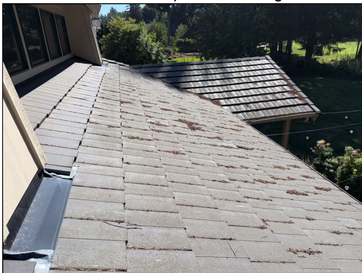
Roof – No Major Concerns
