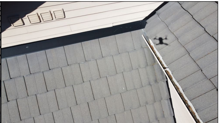
Roof – No Major Concerns
