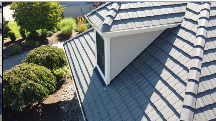
Roof – No Major Concerns
