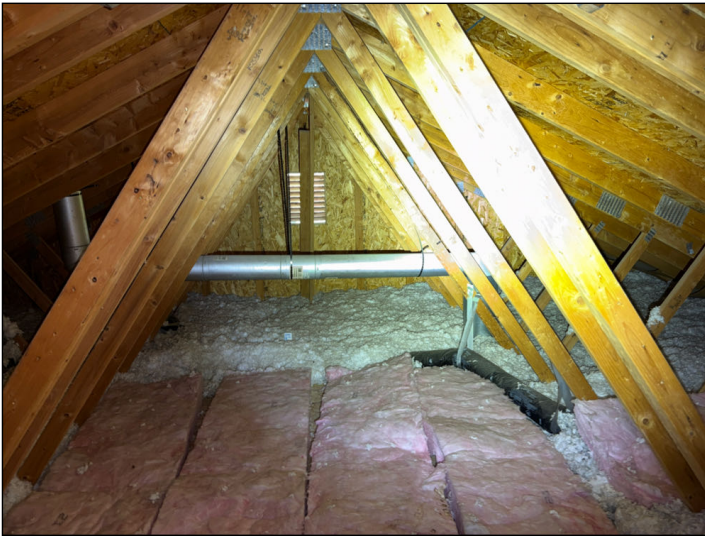
Gable louver vents noted.
