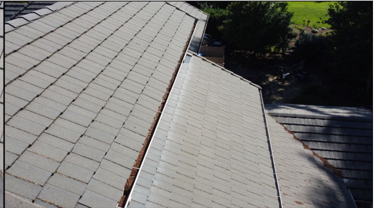
Roof – No Major Concerns
