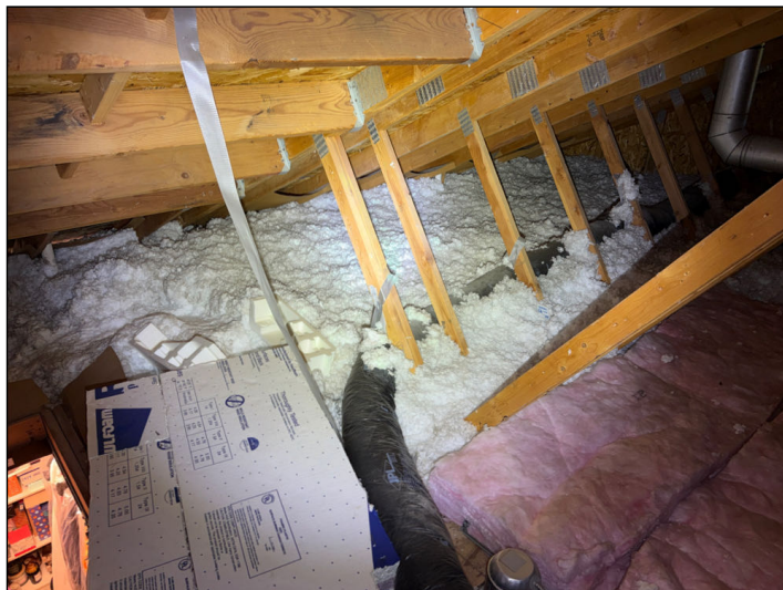
Insulation appears adequate and in good condition.
