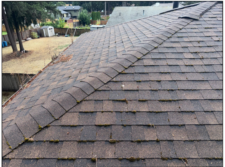
Roof – No Major Concerns
