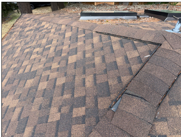
Roof – No Major Concerns
