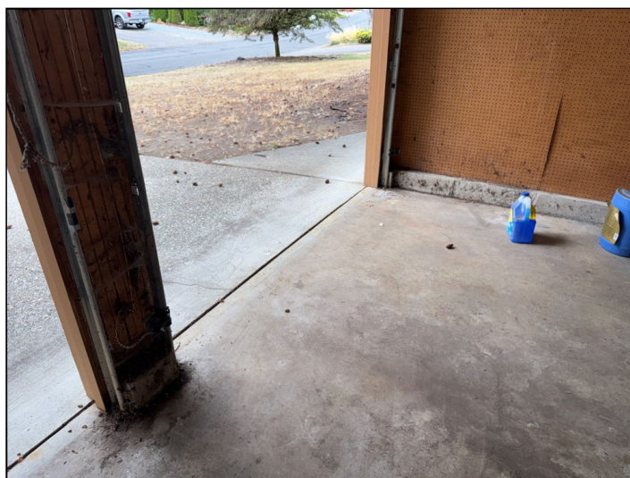
Eye beam system present and operating.
