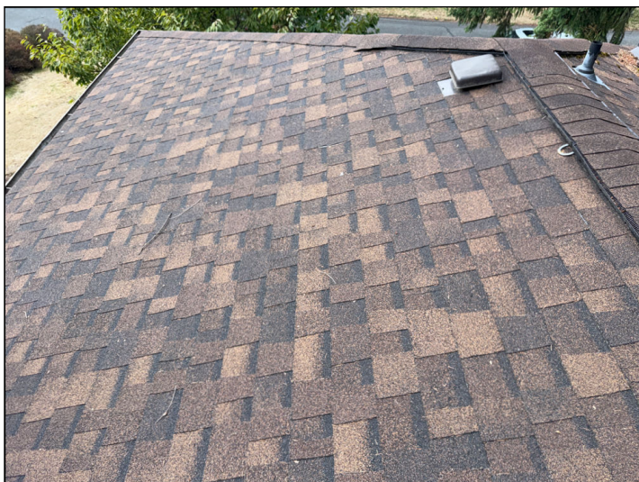
Roof – No Major Concerns
