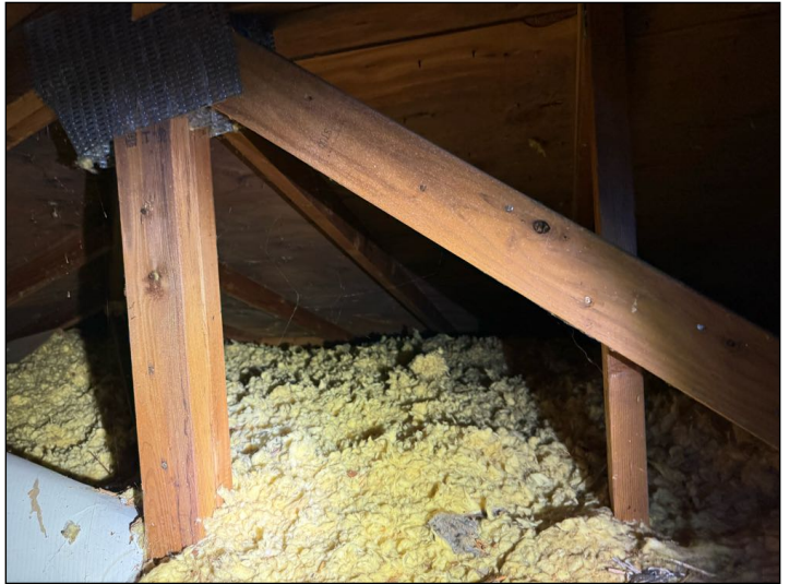
Insulation level in the attic is typical for homes this age. Recommend adding insulation for better home heating performance.
