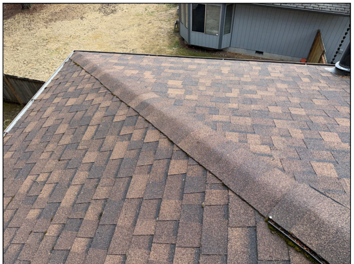
Roof – No Major Concerns
