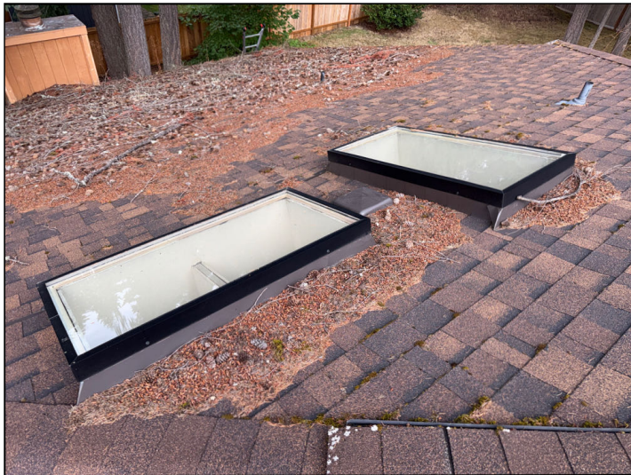
No signs of present or past leaking around the skylight were discovered at time of inspection.
