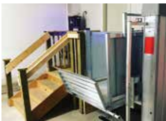
Jessica Evans' EZ-Access Vertical Platform Lift
