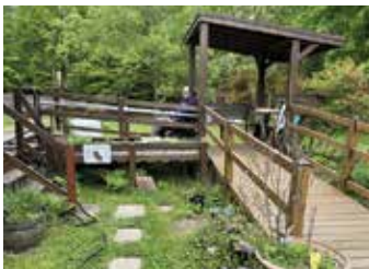
Karen Haley-Wingate's (LGMD R1/2A) exterior entryway ramp with custom high bench seating
