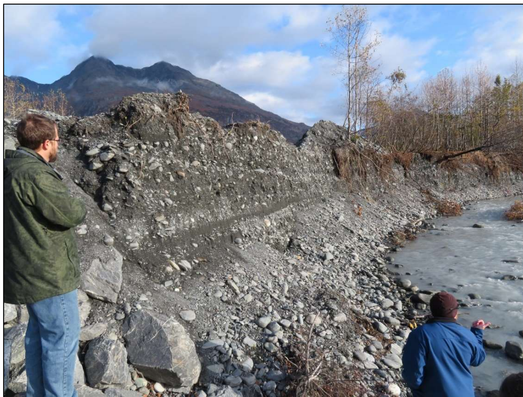
Figure 10. The northern end of west side armored road (Note that it is assumed the alluvial deposits underlie the haul road.)
