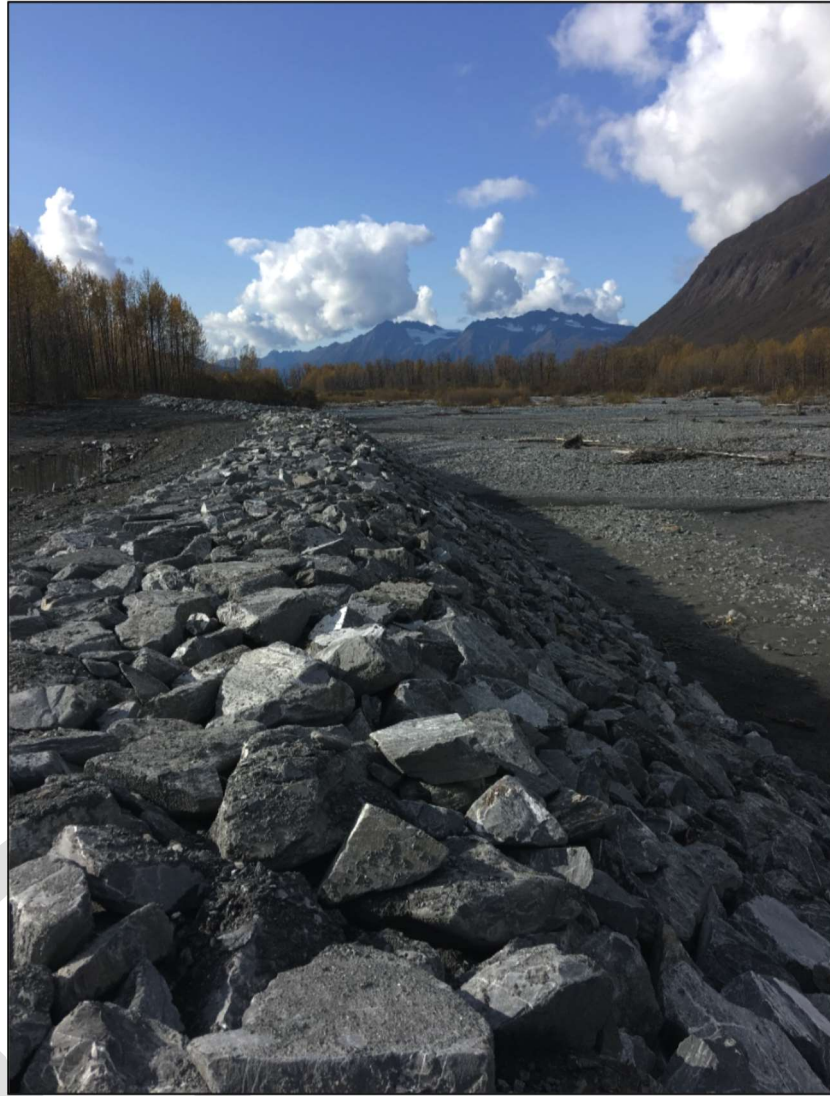
Figure 16: Newly rebuilt and the armored section of the left levee, looking downstream.
