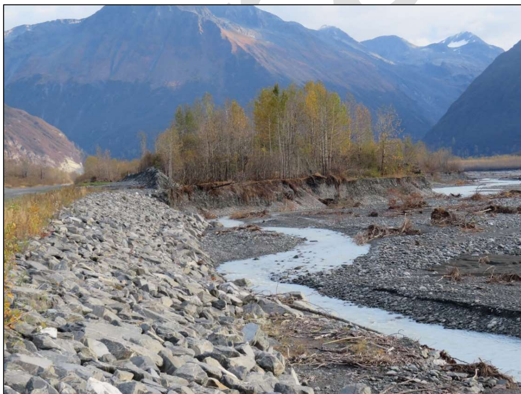
Figure 9. Haul Road armored section near the landfill (Looking north and upstream)
