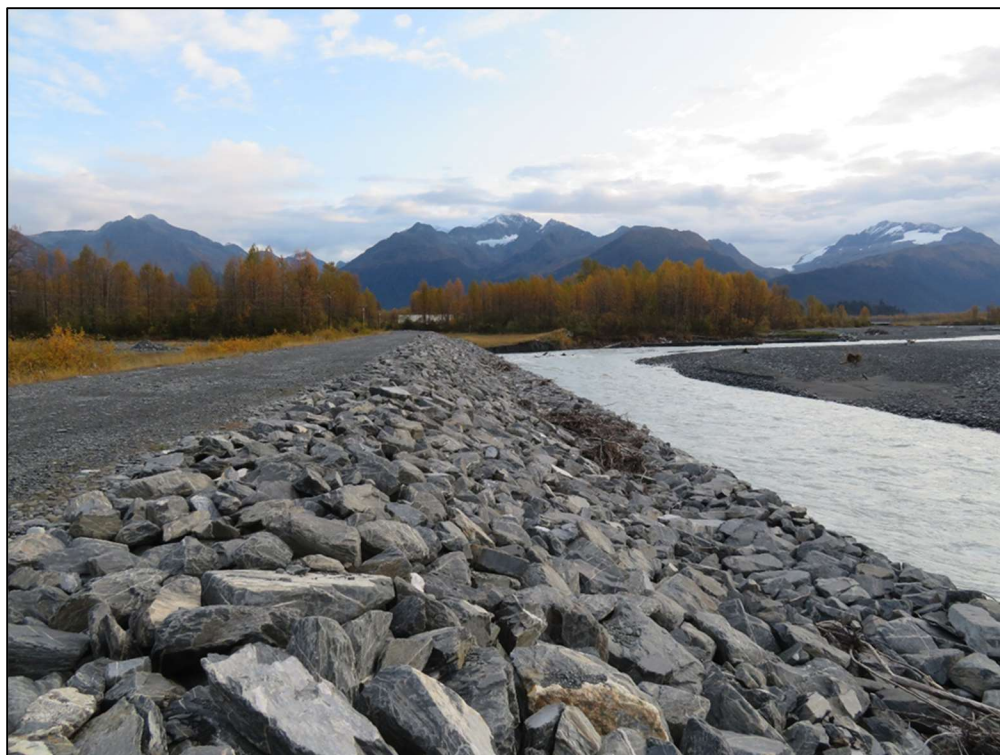
Figure 11. Armored road downstream on the right bank downstream of the Valdez Glacier Stream Bridge #563
