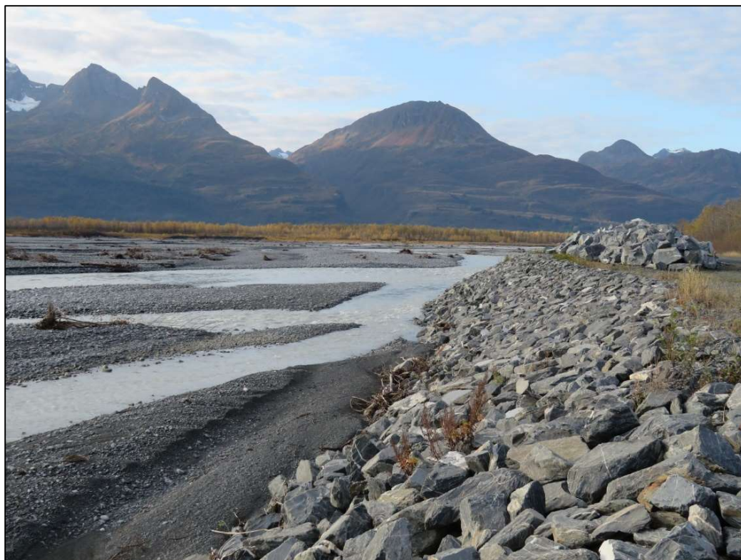
Figure 8. Right bank Training Dike upstream of Valdez Glacier Stream Bridge #556 (Looking downstream toward the bridge).
