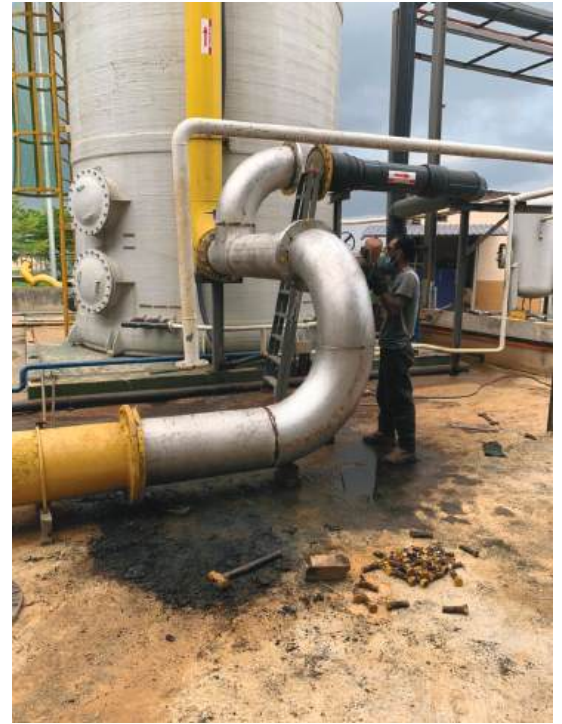
> To Dismantle & Install New Stainless Steel Piping
