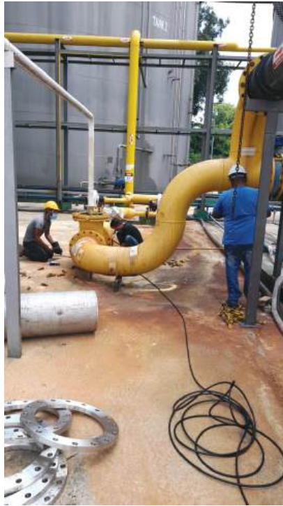
> To Dismantle & Install New Stainless Steel Piping
