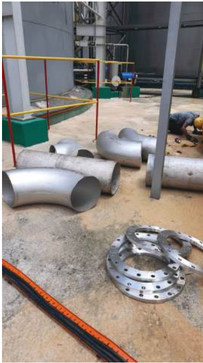
> To Dismantle & Install New Stainless Steel Piping
