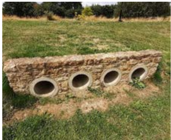
Right: Headwall interconnecting balancing basins at Brimsmore, Yeovil.
