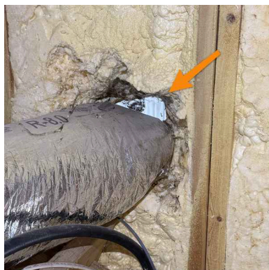
Attic, East Wall
