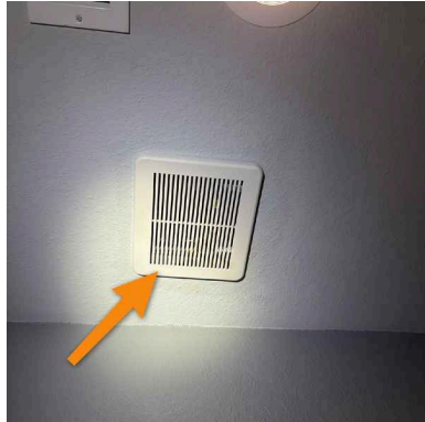
2nd Floor, Bathroom
