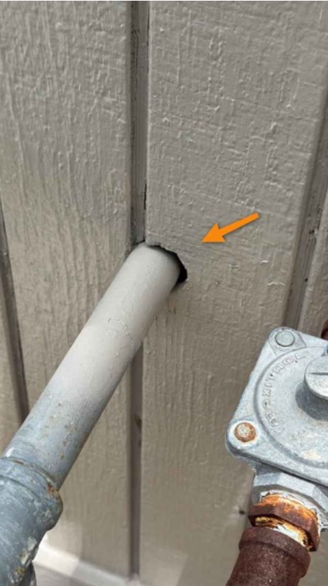
Right Side Of Home. Add exterior sealant.
