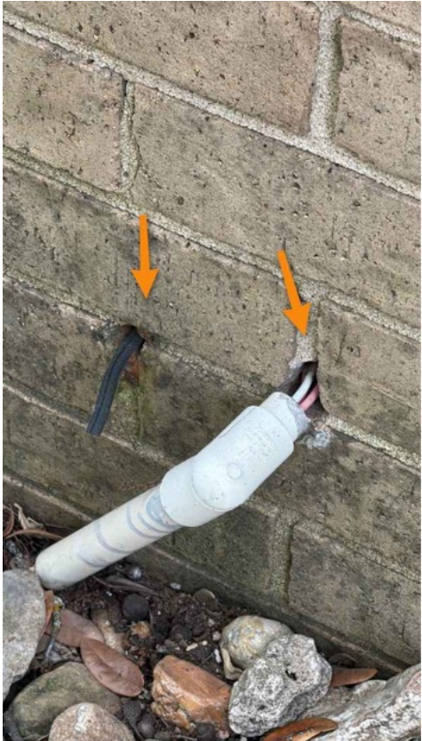
Right Side Of Home. Add exterior sealant
