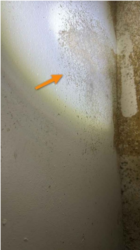
HVAC Closet wall
