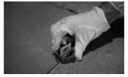
Use the special frame with suction cups to position the slab upon the adhesive bed and tap the slab with the special rubber-coated anti-rebound trowel starting from the center toward the outer sides, in order to ensure complete adhesion and the air outlet. Joints can be grouted after about 2/3 hours in case of fast setting adhesives or after about 24 hours in case of standard setting adhesives.
