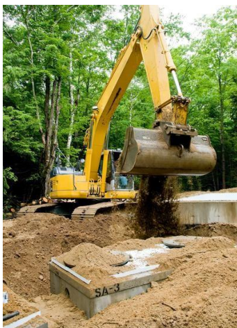
On-site sewage treatment/disposal system installation
