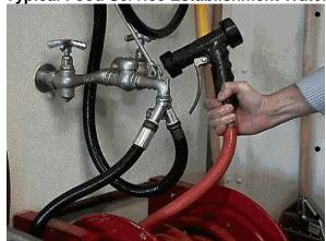
**Pre-rinse or pre-flush hose:** This device is typically located at garbage grinders, mechanical dishwashing machines, and vegetable prep sinks. A spring normally keeps the end of the hose above the sink flood rim level to form an *air gap*. Worn springs allow the end of the hose to fall below the rim.
