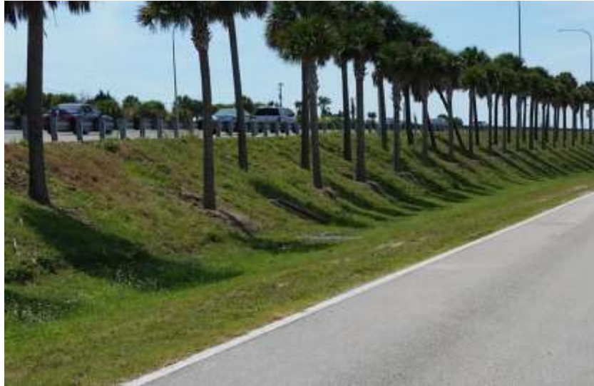
FIGURE 6: WESTBOUND LANE EMBANKMENT OF GANDY BLVD.
