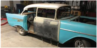
you can then hang the door, and start to locate the new outer rocker. Again, this is a good visual representation of how different the proportions are from a 2-door to a 4-door.
