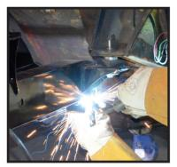
Hold the plate in place and tack on in a few spots, then weld it fully.
