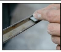
With the clip massaged to proper width, it'll fit in the moulding as it is meant to. This may not be required with all but will be dependent upon the moulding itself.
