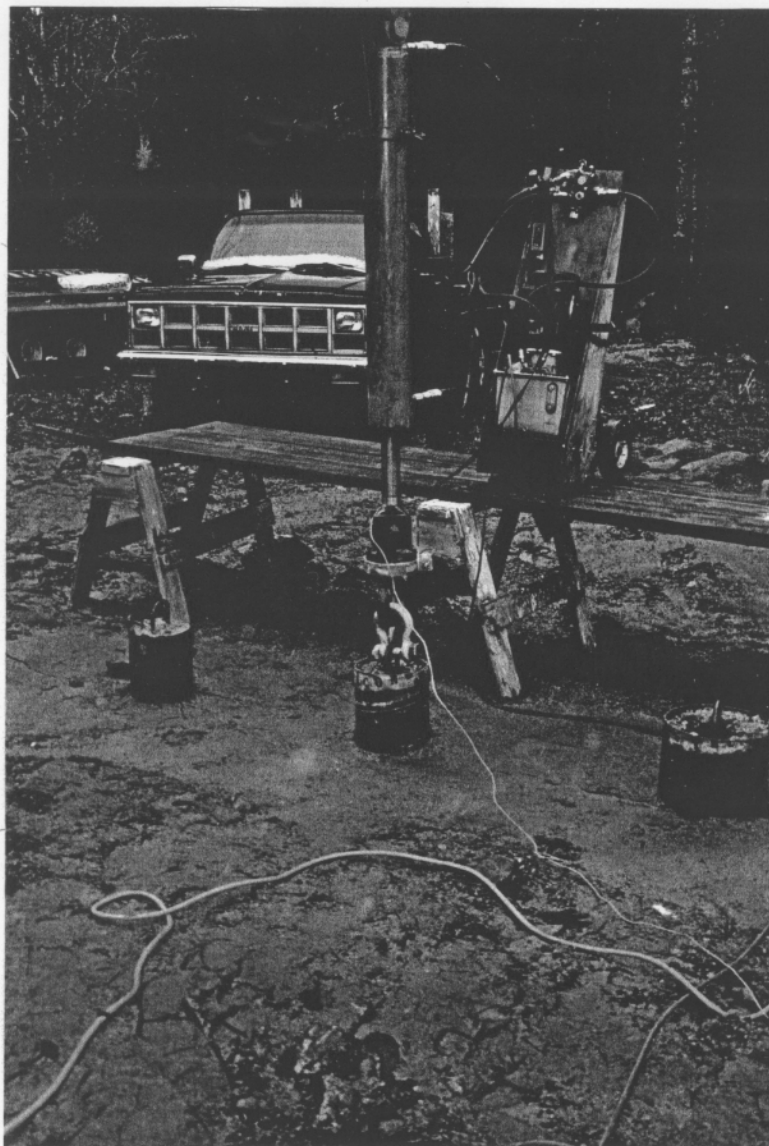
Figure 2: Vertical Load Test Set-up.
