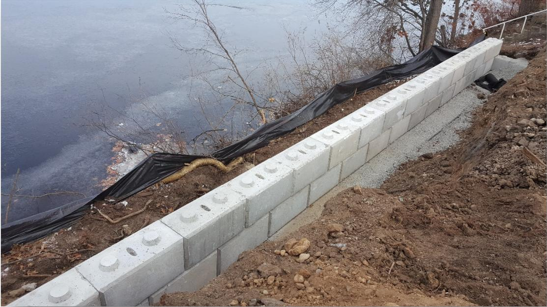
Installation of new retaining wall base blocks using Conigliaro Blocks
