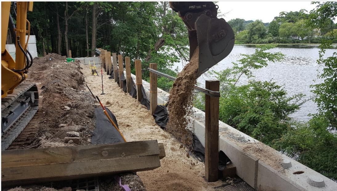
Installation of Guard Rail System
