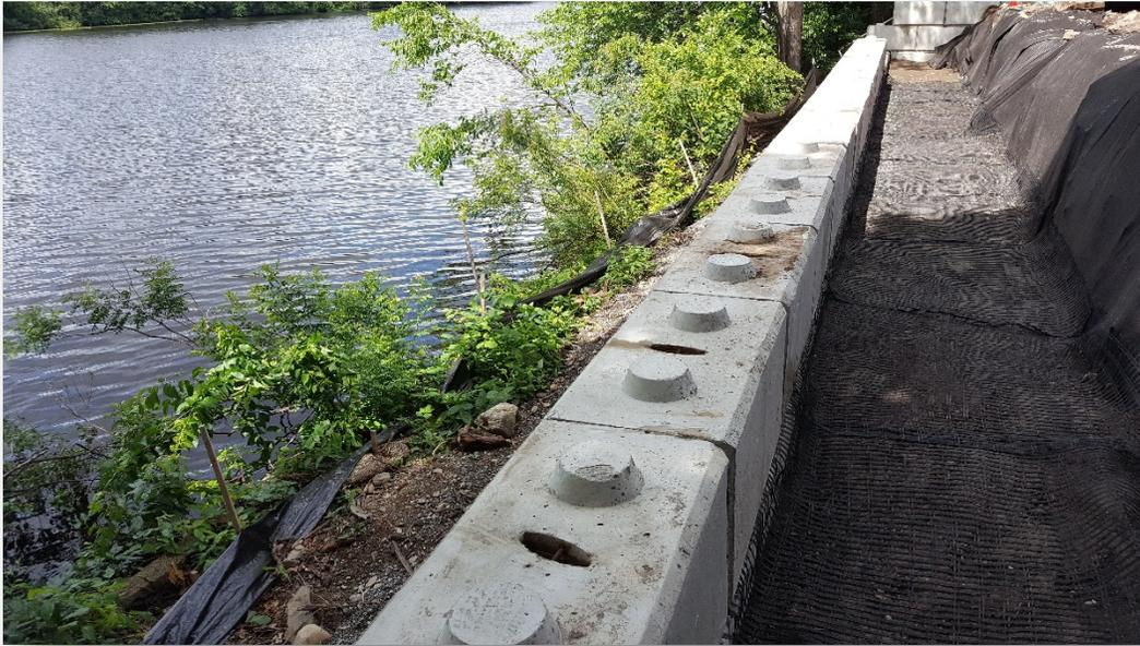
Installation of Reinforcing GeoGrid
