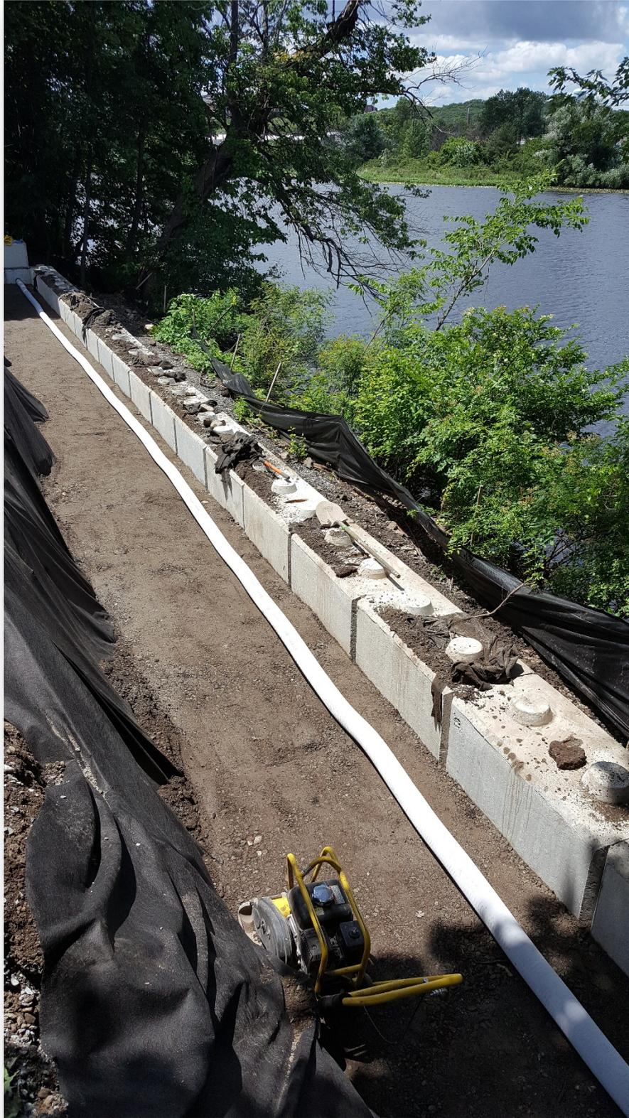
Installation of Behind Wall Drain Pipe
