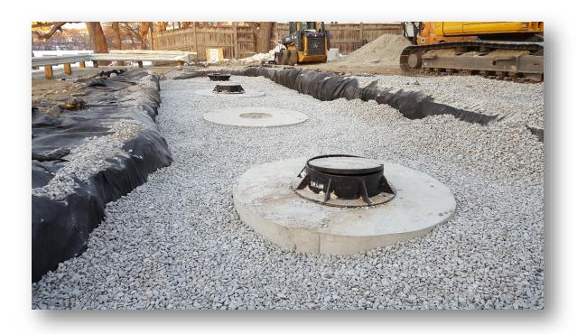
Backfill of leach pit and installation of manhole covers
