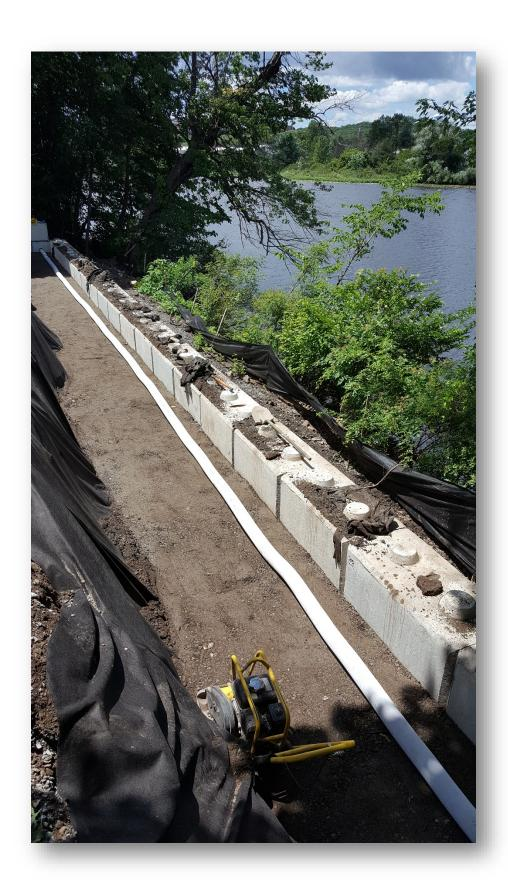
Installation of Behind Wall Drain Pipe
