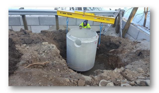
Installation of precast catch basin manholes
