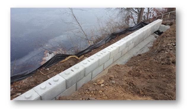
Installation of new retaining wall base blocks using Conigliaro Blocks
