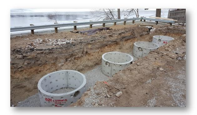
Installation of precast leach pits
