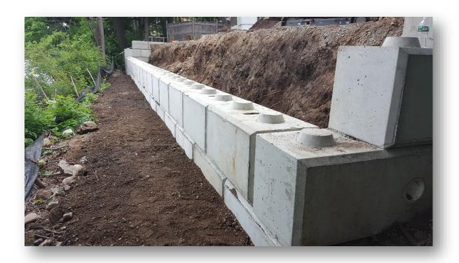
Backfilling of first block
