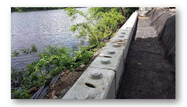
Installation of Reinforcing GeoGrid
