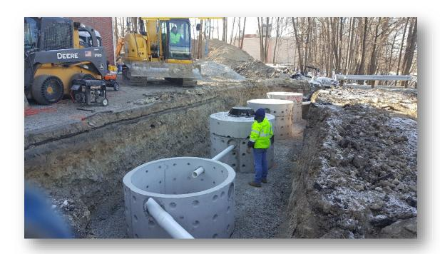
Installation of below grade connecting piping
