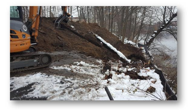
Demolition of failing creosote timber wall within two feet of the river
