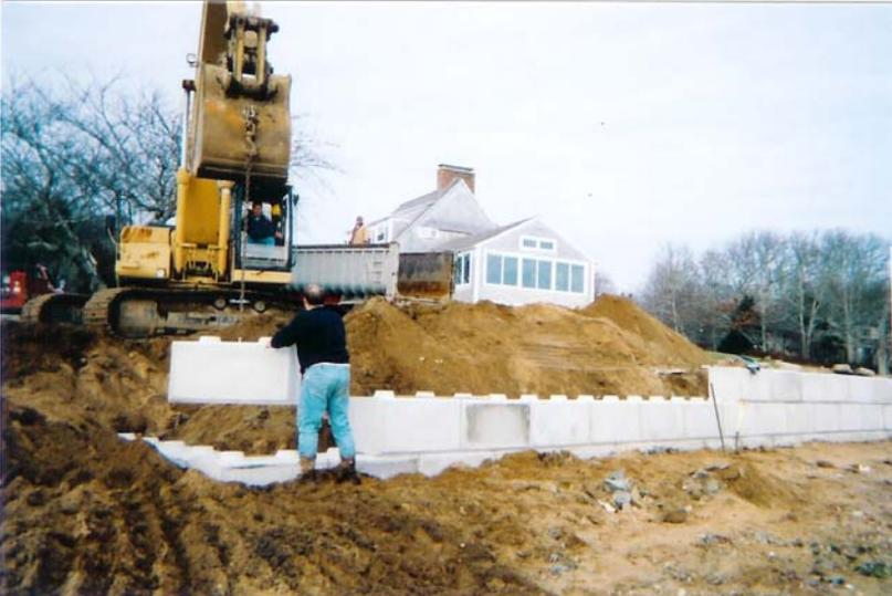
*We offer Plus-Crete and Standard Concrete Blocks with interlocking knobs, perfect for Seawalls subjected to tidal pressures!*
