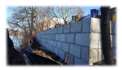
When dealing with blocks with a designer finish, we pour a special Inside Corner Block which is shown here:
