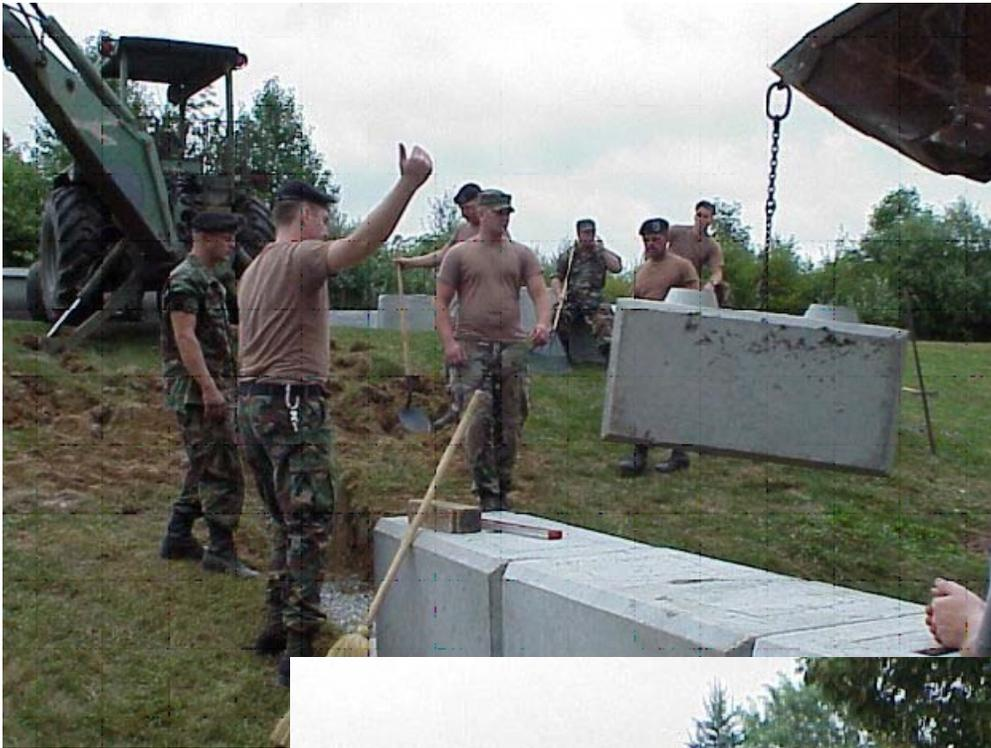
*This main gate was hardened with a 4 ft high Plas-Crete Force Protection Block Wall designed to slow and channel vehicles towards the security check point.*
