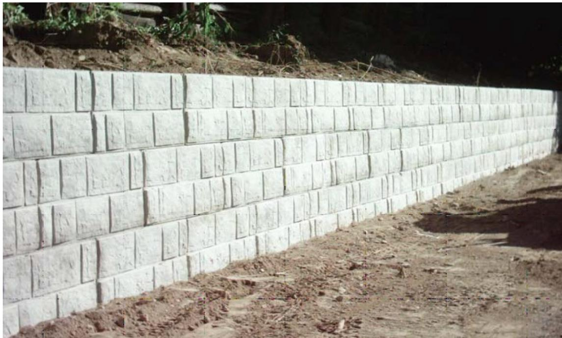
*Protective Earth Berm retained by Plas-Crete Force Protection Blocks with Cut Stone Designer Finish. Once the berm is planted, this aesthetically pleasing force protection solution is complete!*
