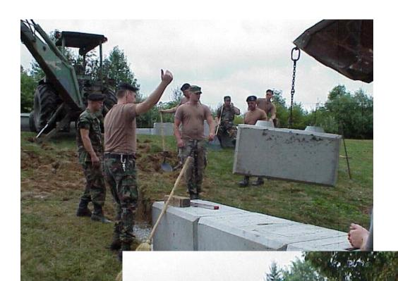
This main gate was hardened with a 4 ft high Plas-Crete Force Protection Block Wall designed to slow and channel vehicles towards the security check point.
