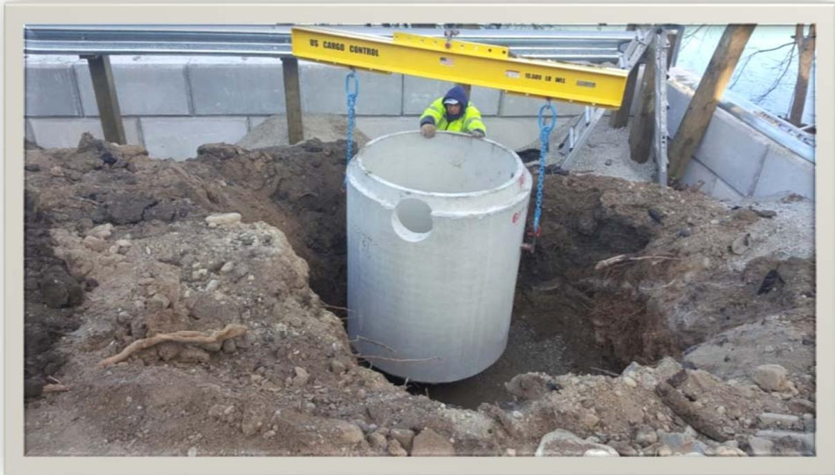
Installation of precast catch basin manholes
