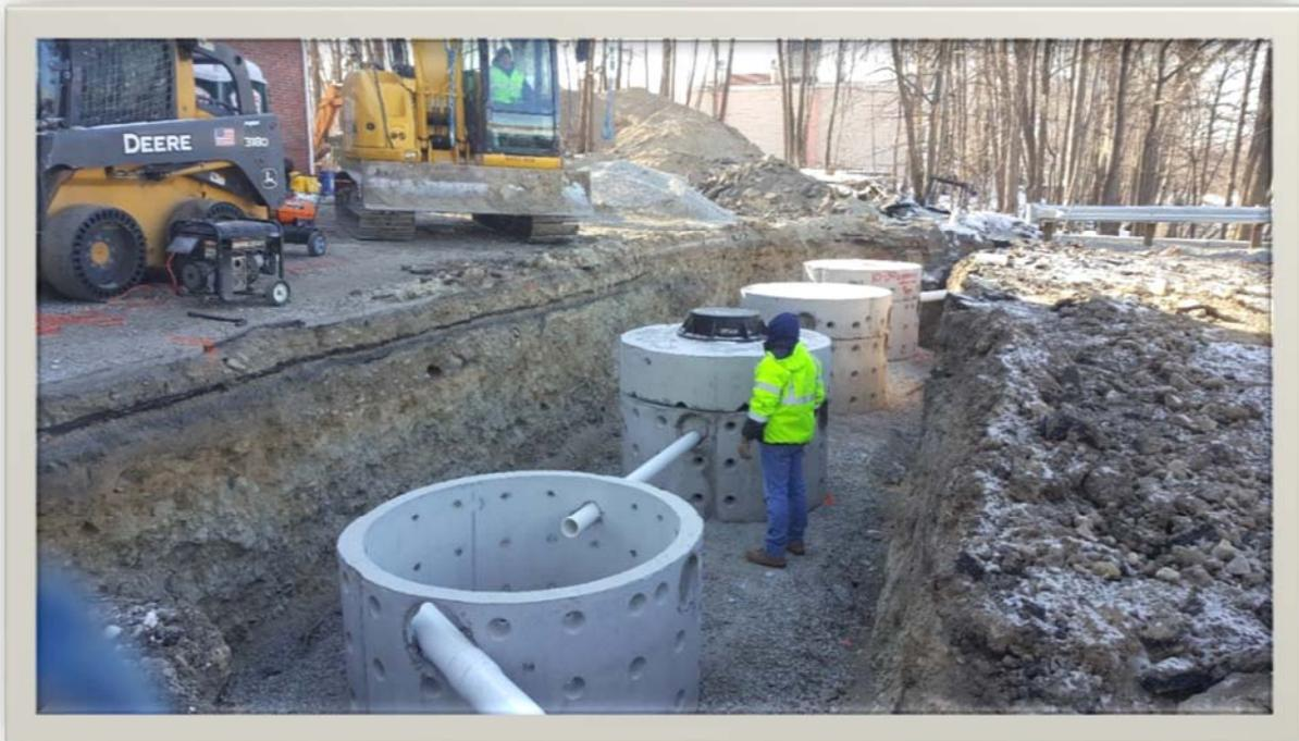
Installation of below grade connecting piping
