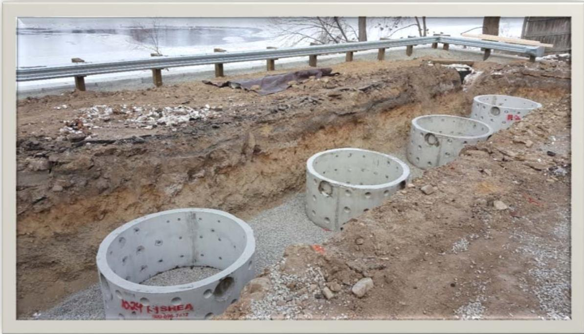
Installation of precast leach pits
