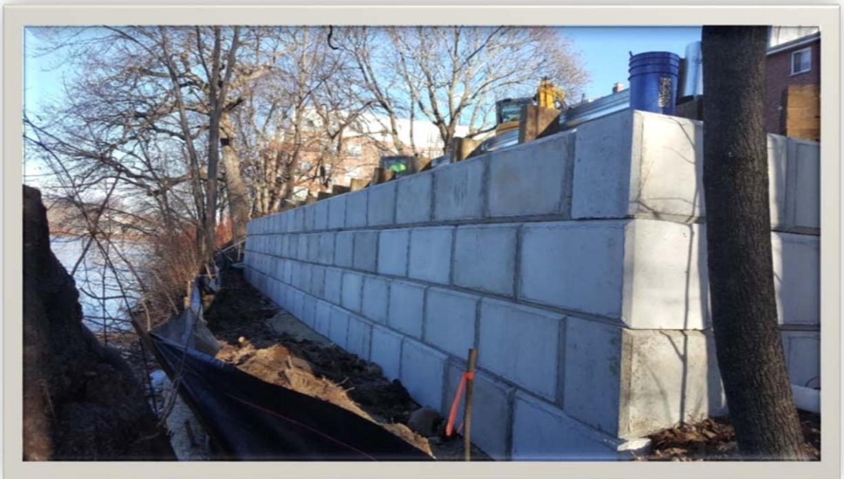
Completed retaining wall using Conigliaro Blocks
