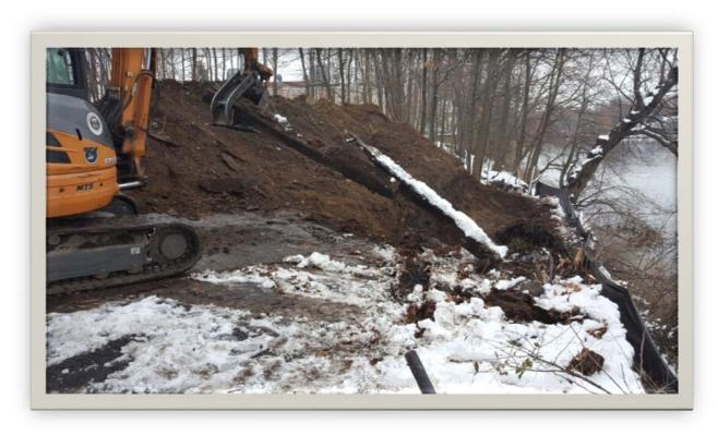
Demolition of failing creosote timber wall within two feet of the river
