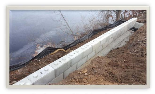
Installation of new retaining wall base blocks using Conigliaro Blocks
