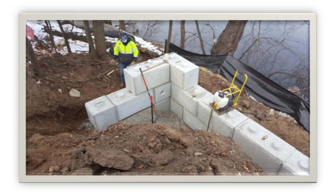
Installation of wall corner and pipe penetrations blocks using Conigliaro Blocks
