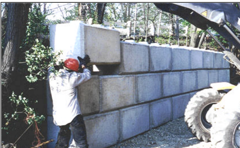
Placing Plas-Crete block
