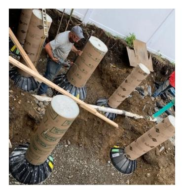
Filled with 4000 psi concrete and vertical rebar(s) for added tensile strength.
