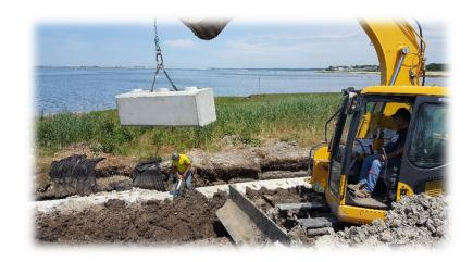
Blocks weigh 1000 to 4000 pounds each, so it is imperative that the onsite contractor have the proper lifting gear to safely unload the blocks.
