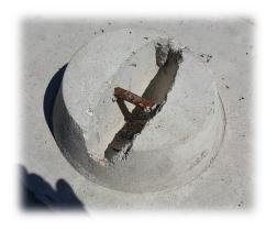
This pick point is centered on the top of each block, i.e. for full knob blocks the pick point is between the knobs and for a half knob block the pick point is within the knob.
