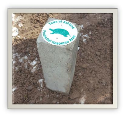
Conigliaro Block manufactures and installs permanent concrete No-Disturb markers along wetland buffer zones as required by many Conservation Commissions in Massachusetts.
