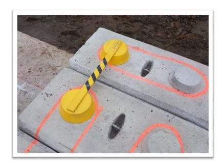
Conigliaro Block shall provide a loaner Block Placement Gauge if requested by the installer. This gauge is useful to insure blocks, and their male knobs, are placed in proper alignment such that future blocks fit, and sit, properly.
